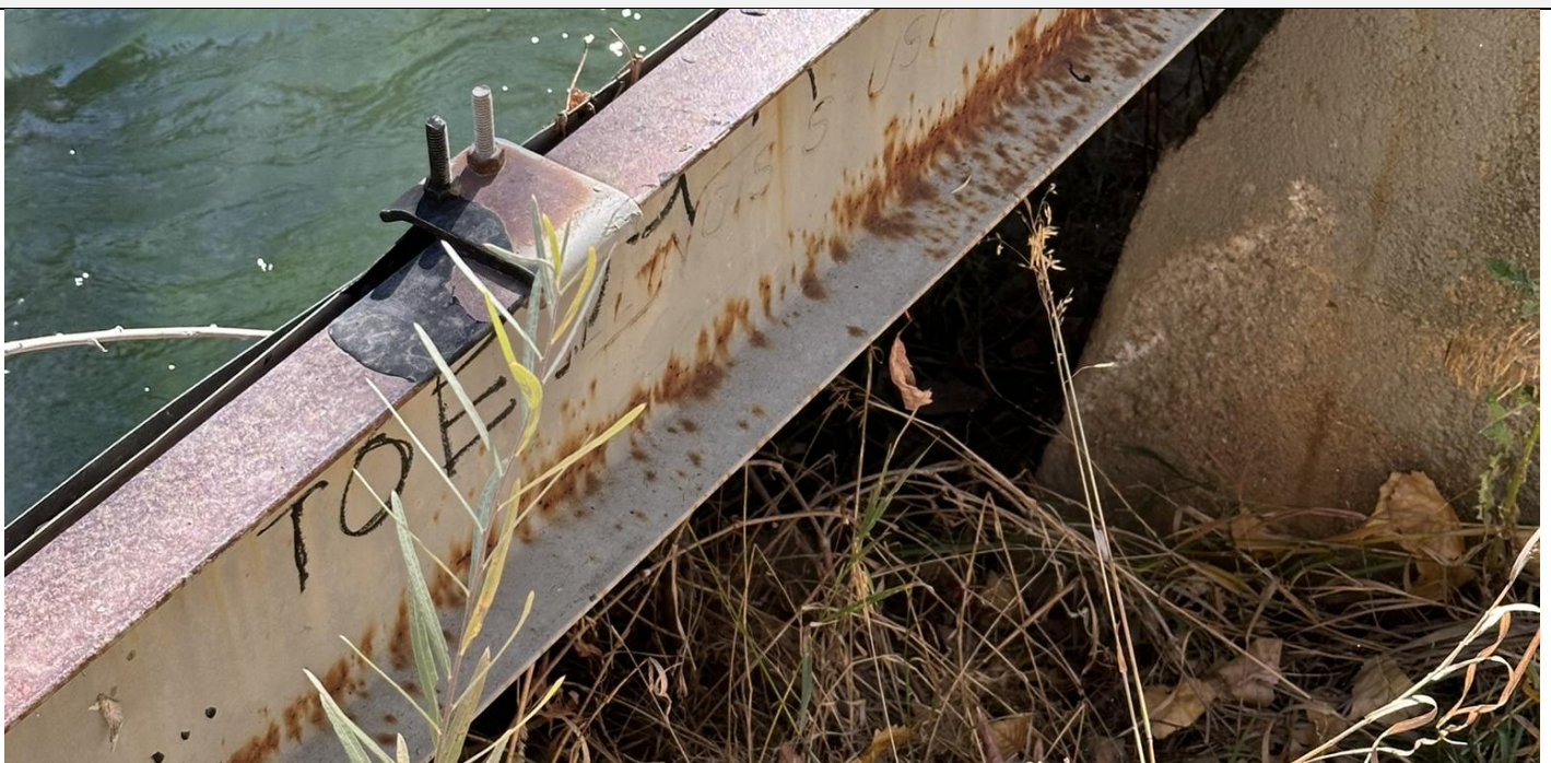
Close-up of a girder. Negative
