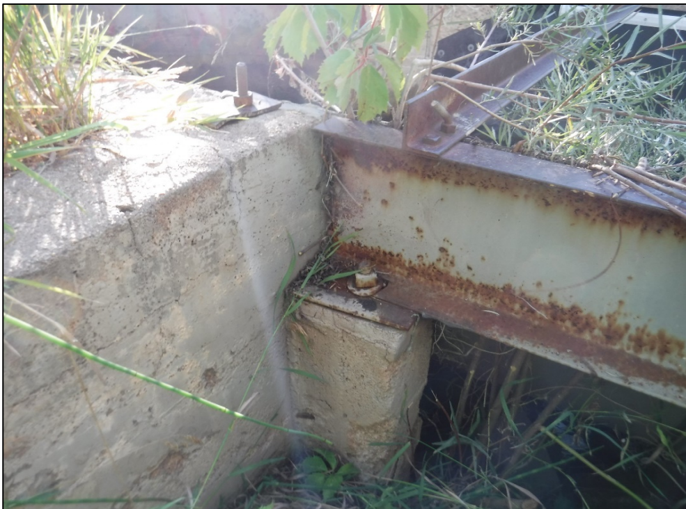
Northwest bearing between beam and abutment.
