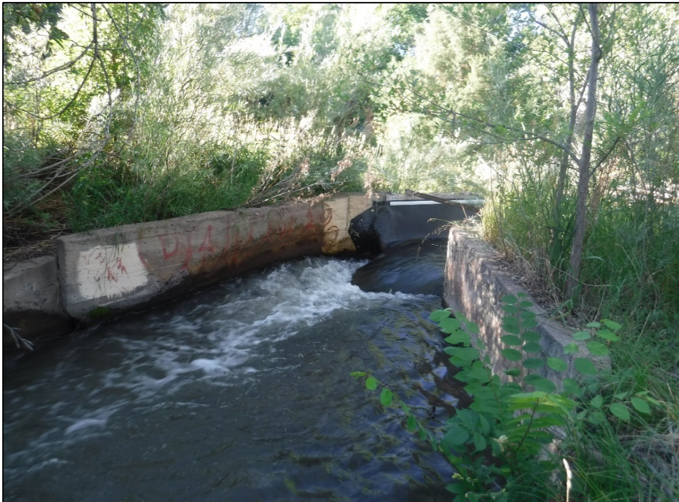
Flume looking southwest.
