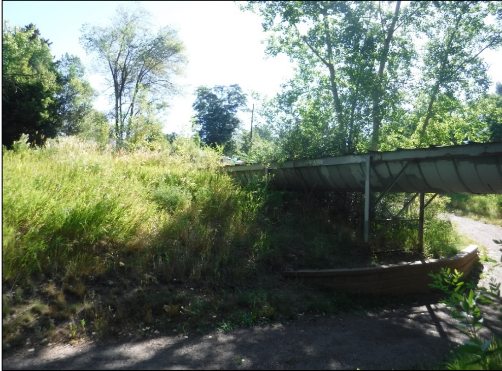
Elevation looking northeast towards Abutment 14.
