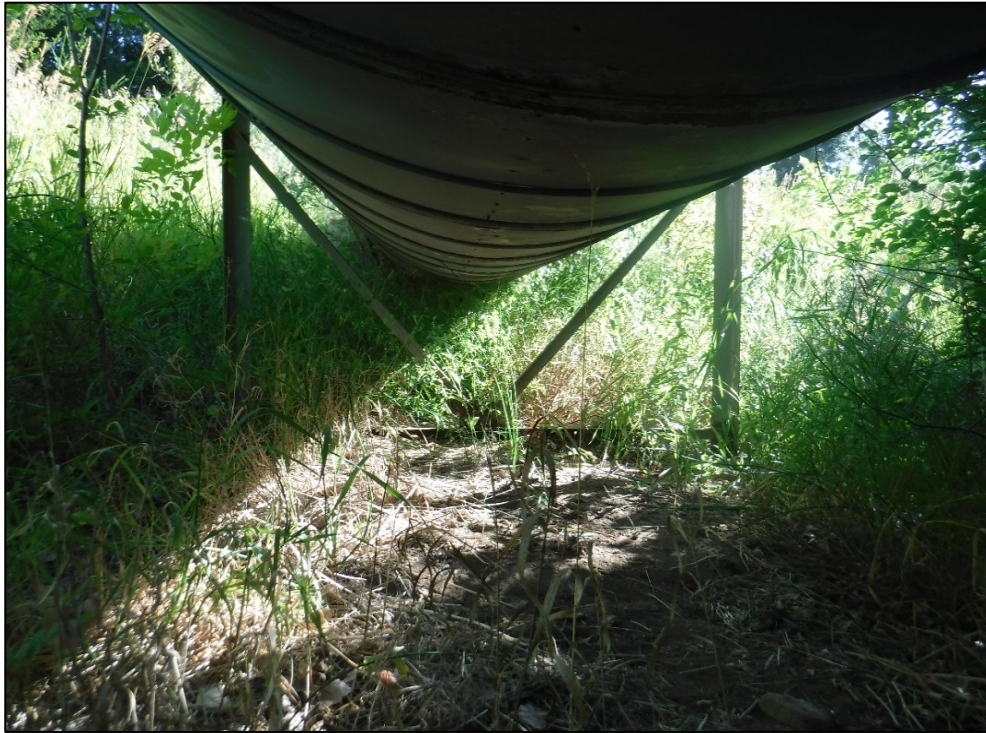
Pier 12 trestle general.
