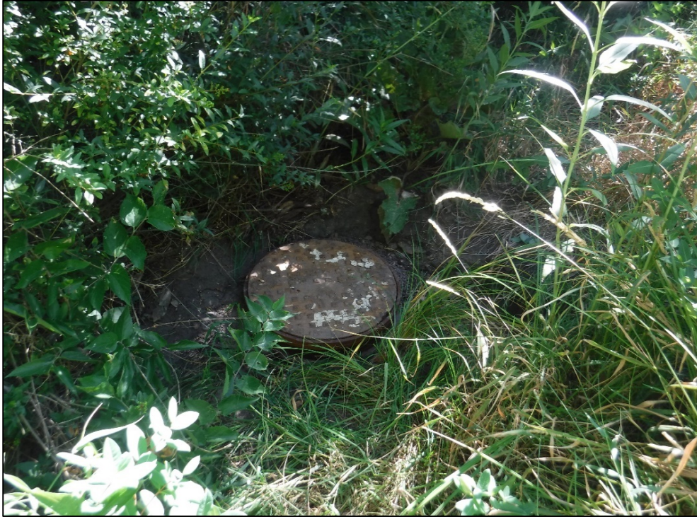
Storm drain at east side of Pier 5.
