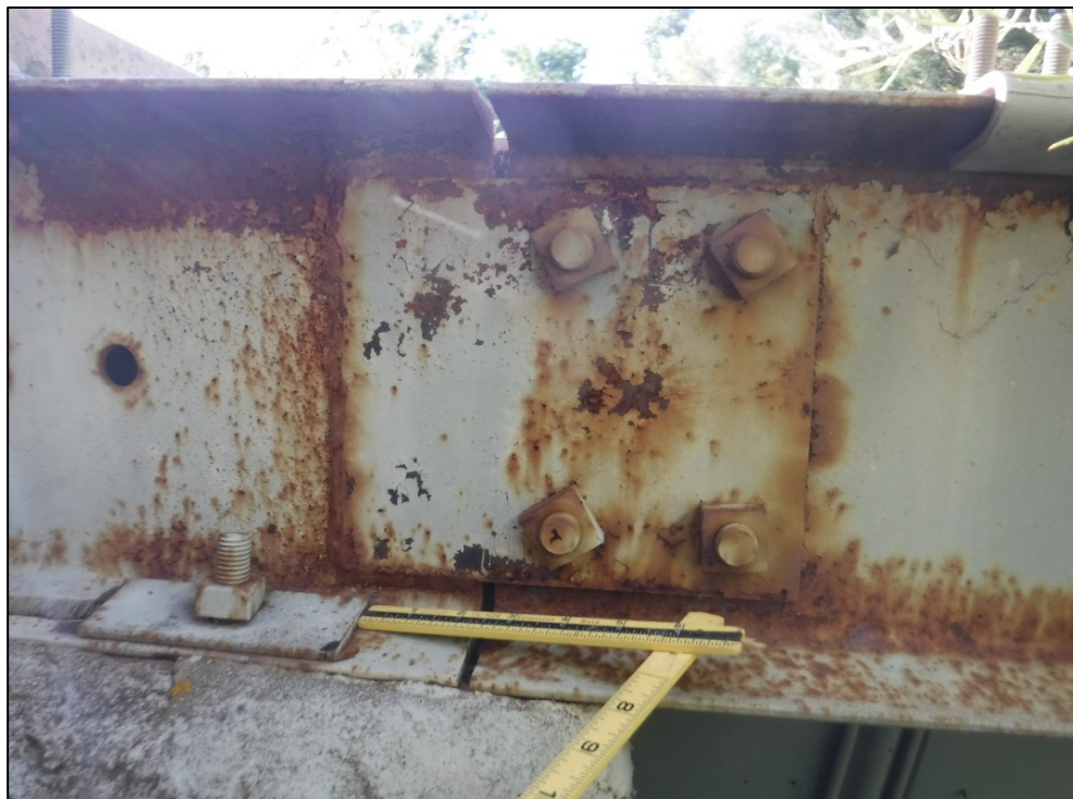
Beam web splice connection at Pier 13, typical.
