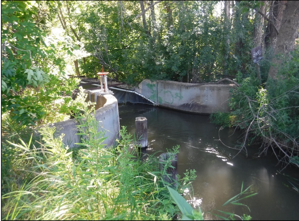
Flume looking northeast.
