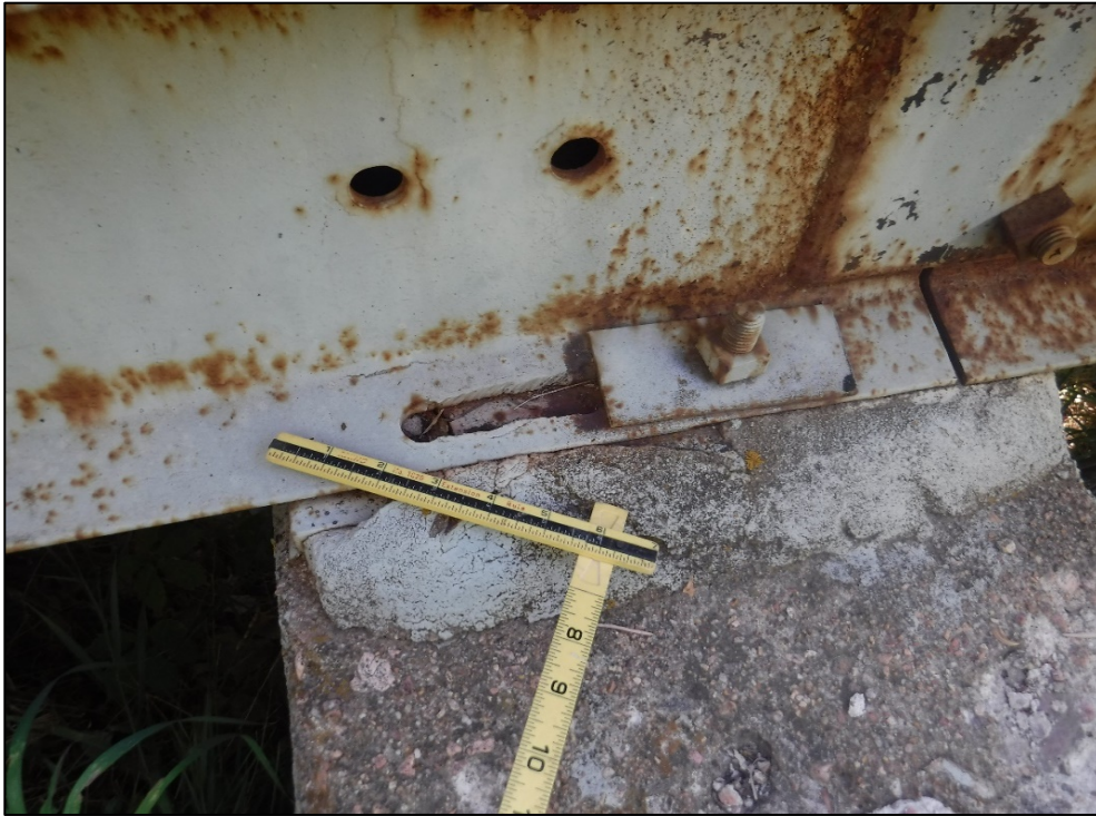
Moveable bearing at Pier 13, typical.
