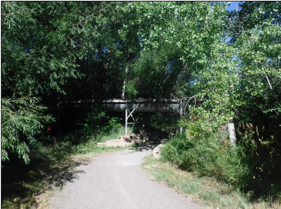
Elevation looking west (Spans 8, 9, and 10).
