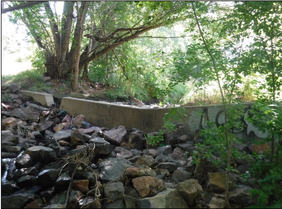
Concrete weir across channel under Span 6.
