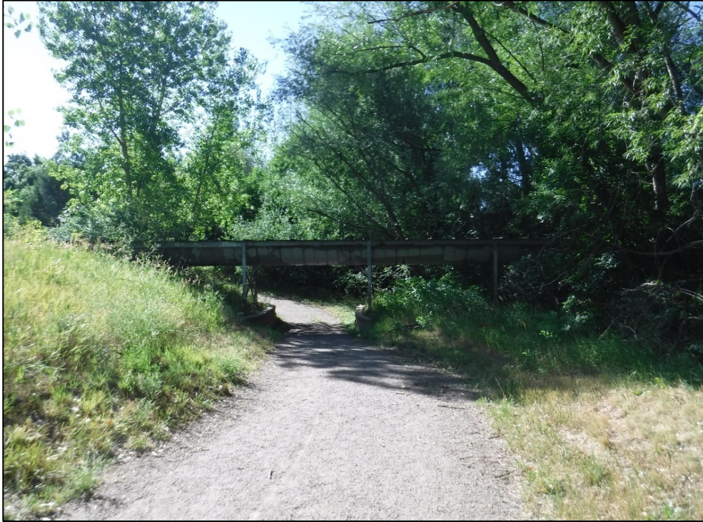
Elevation looking east (Spans 8, 9, and 10).
