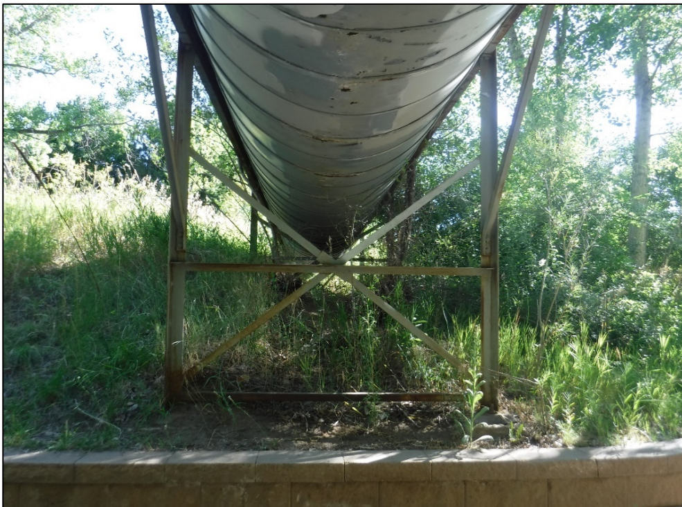
Pier 10 trestle general.
