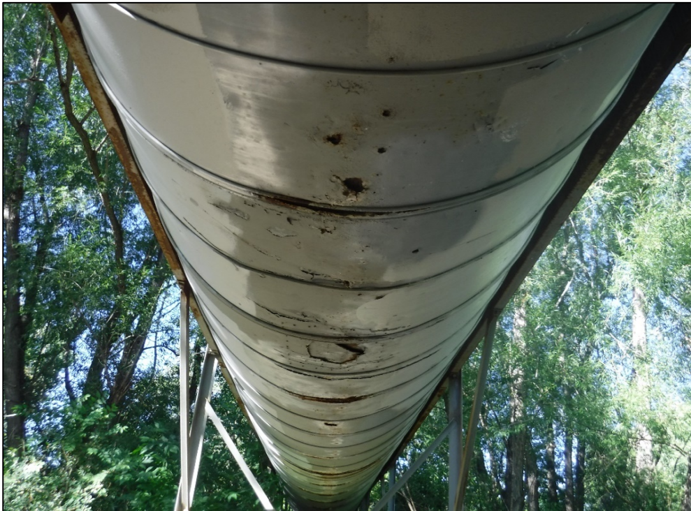
Span 9 underside looking north.
