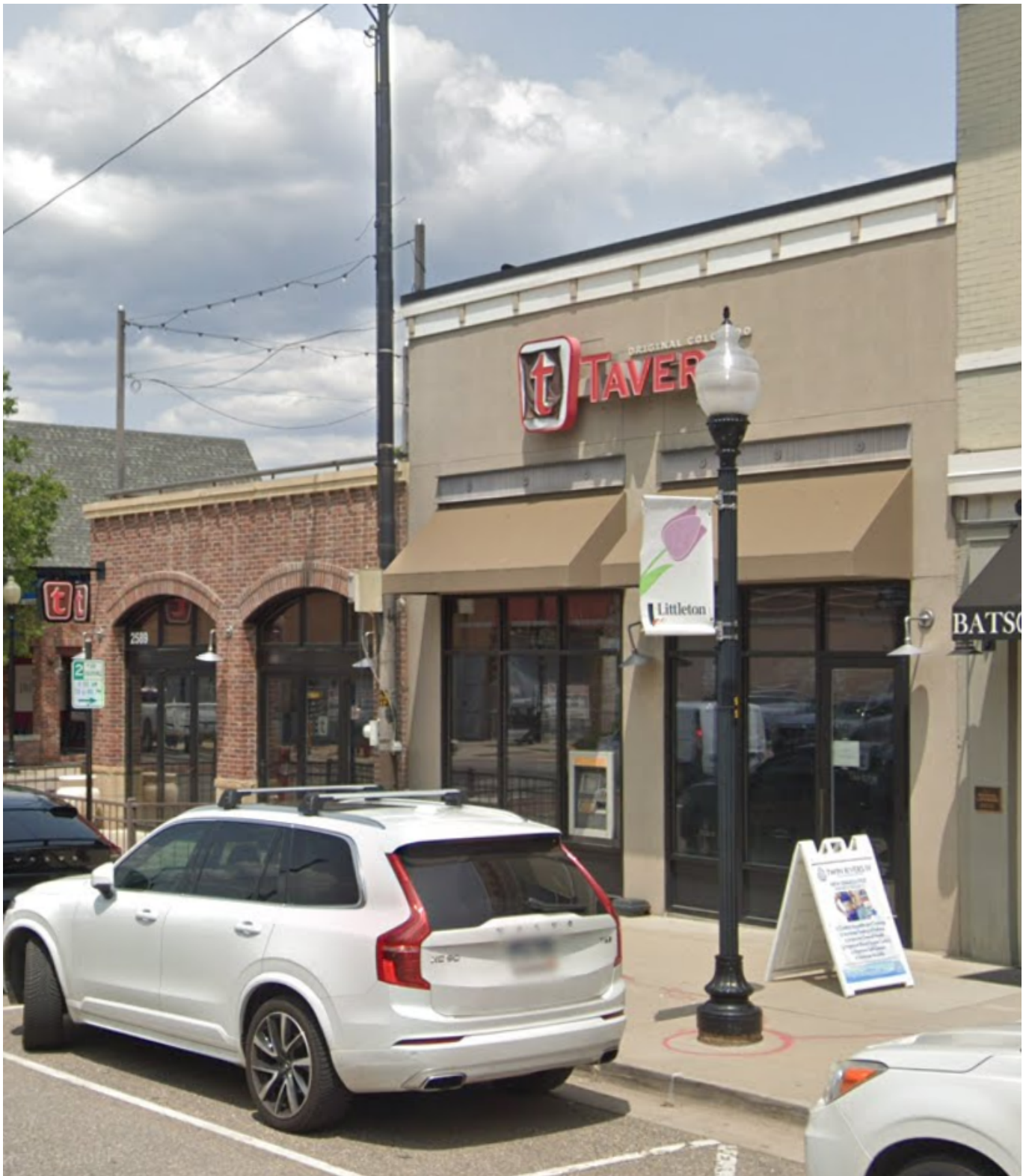
2589 W. Main Street View from Southwest - As Built
