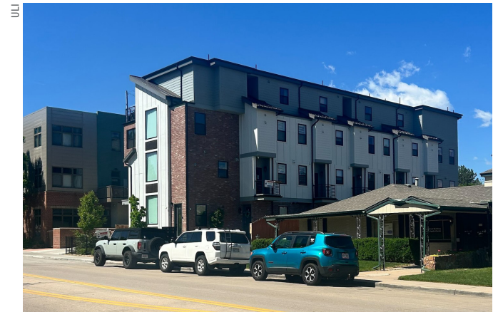
Nearby residential on Prince
