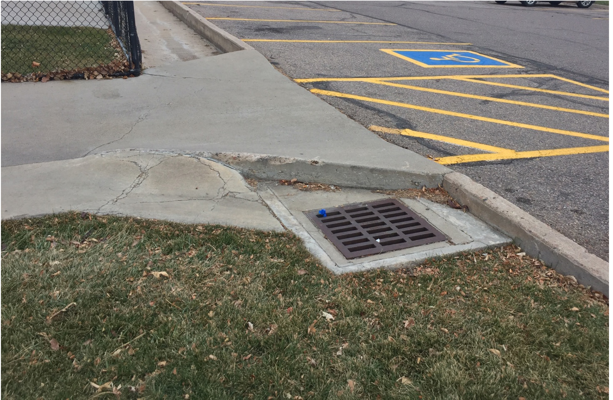
Image 11 - Accessible ramp at parking lot, images illustrates lack of detectable warning strip and cracked concrete.
