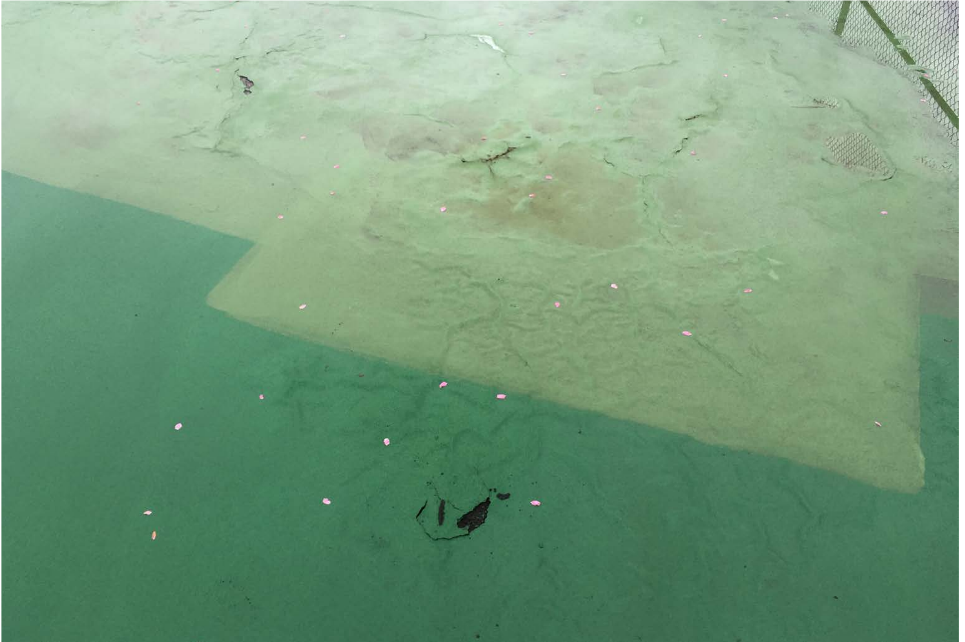
Image 9 - Tennis Court Surfacing - photo illustrates cracks forming in asphalt and crack seal coating since previous repairs.
