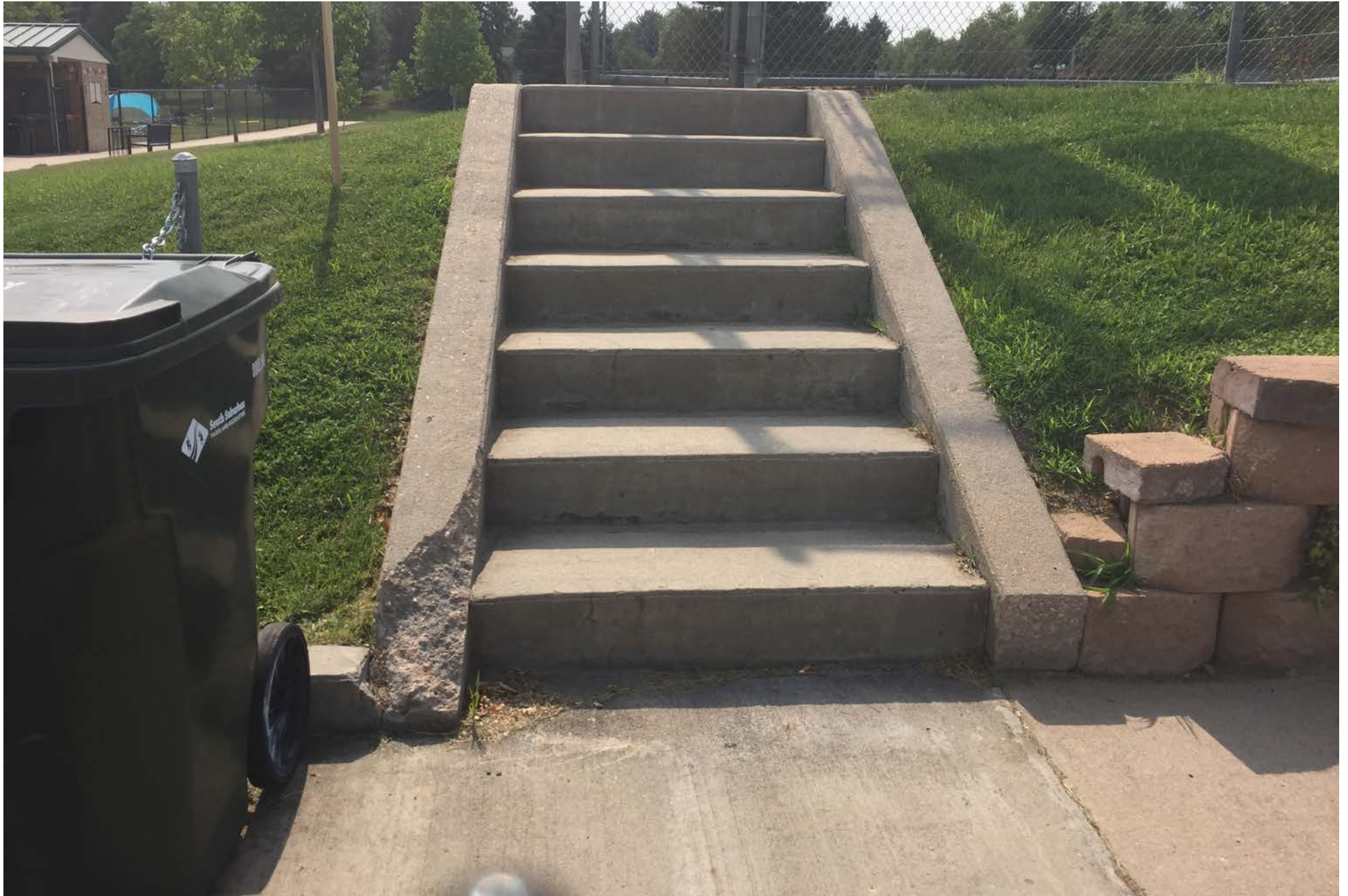
Image 10 - Condition of stairs to tennis courts. Retaining wall at the right needs replacement stones.
