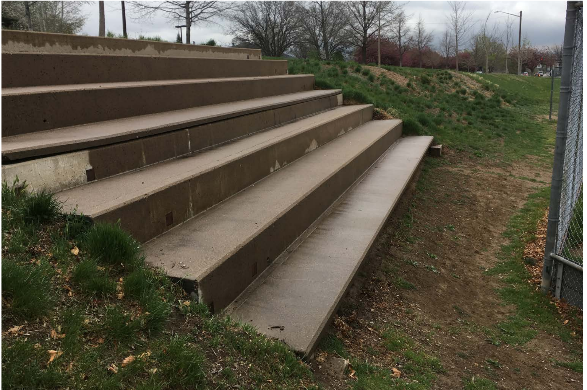
Image 3 - Northern ballfield - concrete bleachers, photo illustrates steep cross slopes, lack of accessible access and lack of accessible seating.
