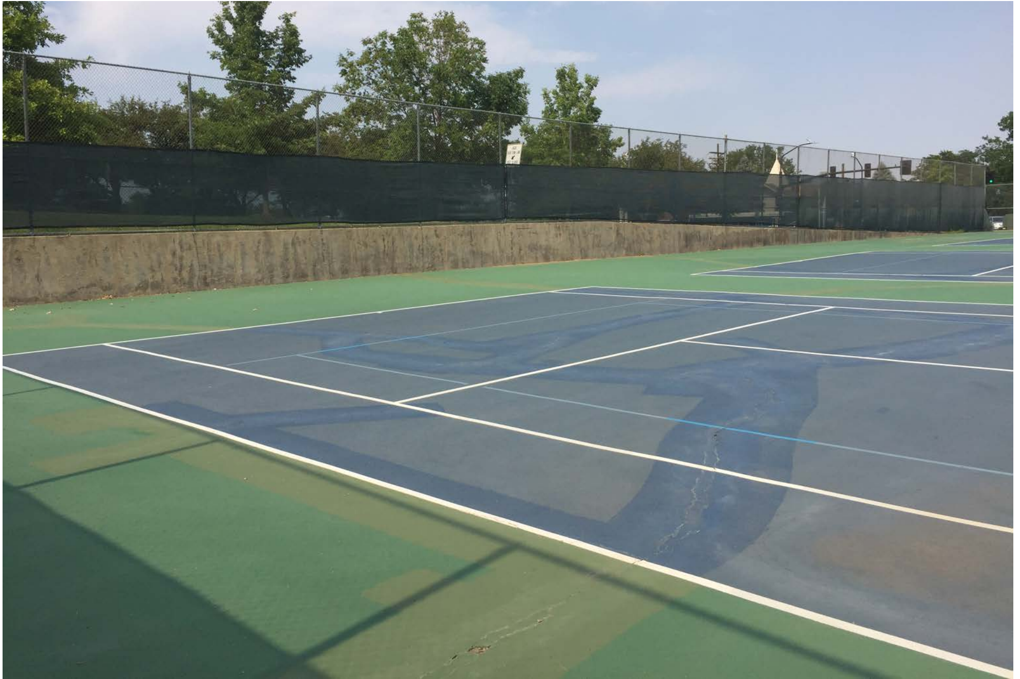
Image 8 - Tennis Court Surfacing - examples of cracks forming since previous years repair, previous repairs, and current condition of the existing asphalt surfaced courts.
