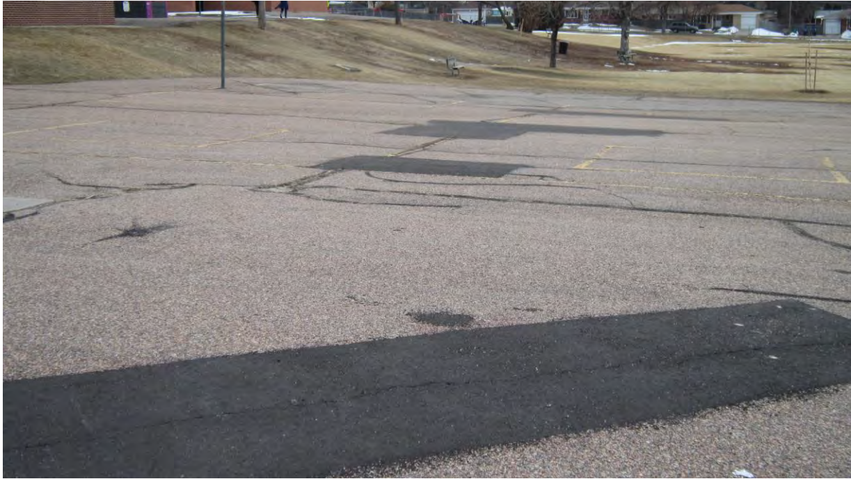
Uneven surface with cracks and ridges.
