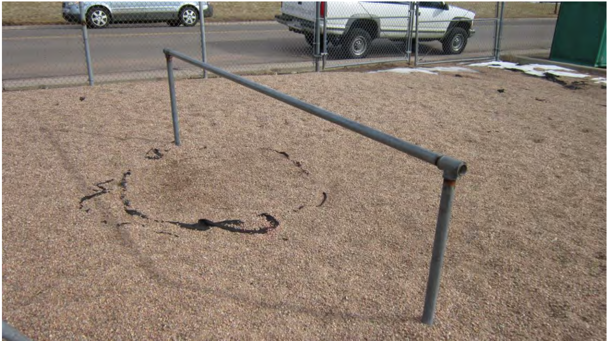
Close-up of metal play structure. Rusted and missing end pieces.
