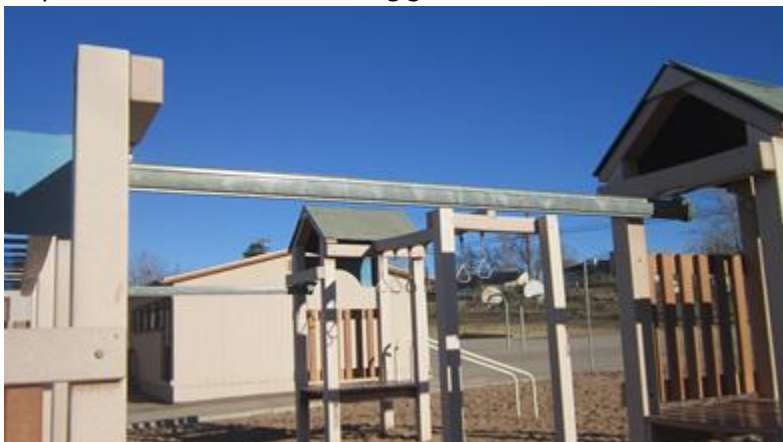
Play Structure in 3-5 with missing glide bar
