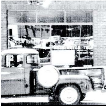
The original windows had three fixed transom windows above two larger fixed panels
