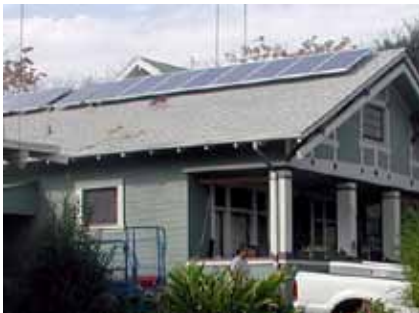
Mount collectors flush below the ridgeline on a sloping roof.
