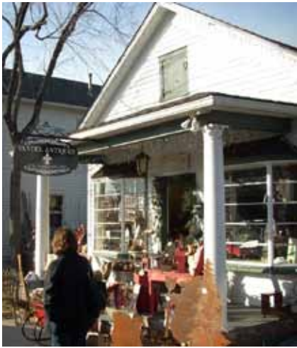
The adaptive reuse of this residential structure to commercial uses maintained the historic character of the property while accommodating the new function to keep it in active use.
