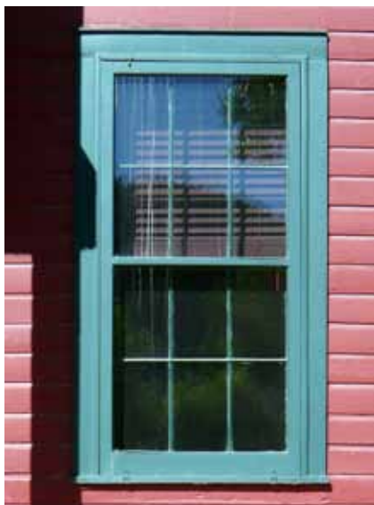
Consider use of a storm window to enhance the energy efficiency of an existing historic window.
