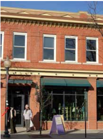
This commercial building in Downtown Littleton has many typical elements of a storefront (see diagram at left).
