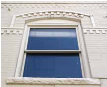
The character-defining features of a historic window, its distinct materials and its placement should be preserved.
