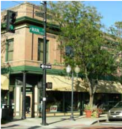
The Coors building, located within the Opt-in Main Street Historic District, has double-hung windows and awnings; both are example of historic building features used for energy efficiency.
