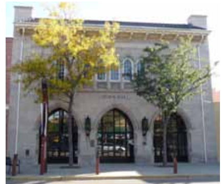
The Old Town Hall serves as an accent to the traditional commercial storefront framework of the historic district. The building has a row of three gothic arches defining the street level, with a wall of recessed doors and windows.
