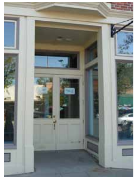
The character-defining features of a historic door, its distinct materials and placement should be preserved.
