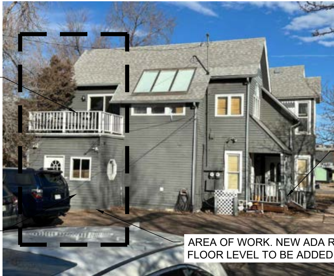
CURRENT PHOTOGRAPH SOUTH ELEVATION LOOKING NORTH
