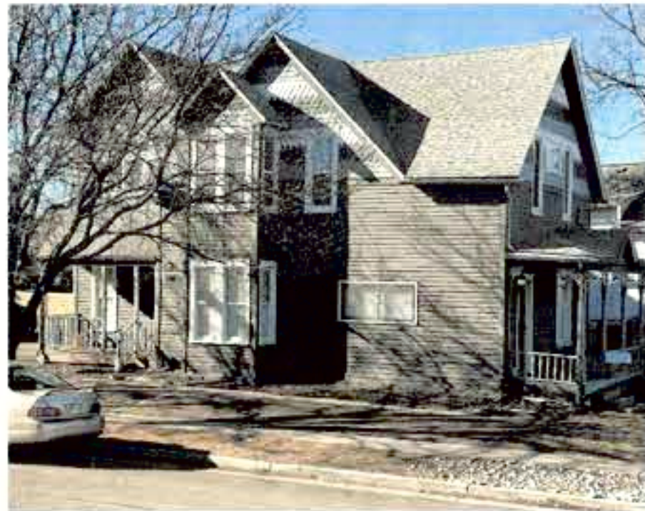
CURRENT PHOTOGRAPH EAST ELEVATION
