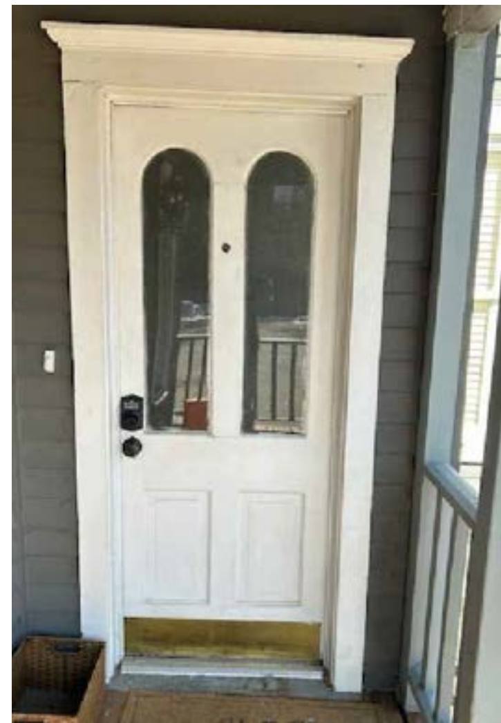
CURRENT PHOTOGRAPH EAST DOOR EXTERIOR
