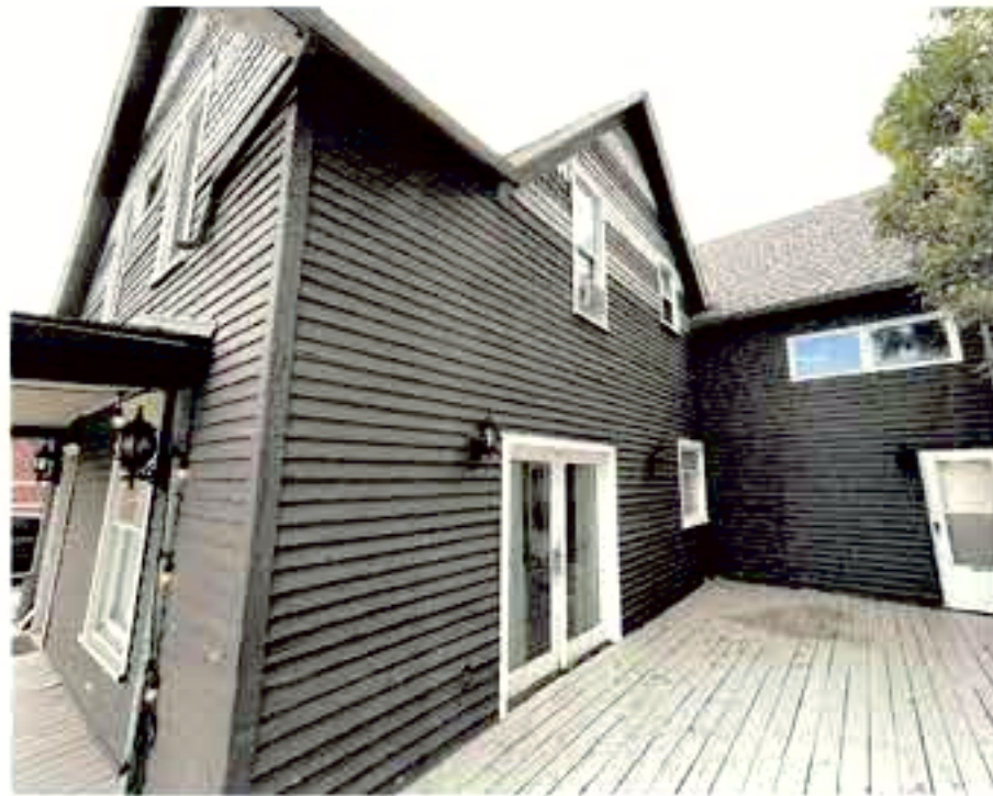
CURRENT PHOTOGRAPH DECK - WEST SIDE
