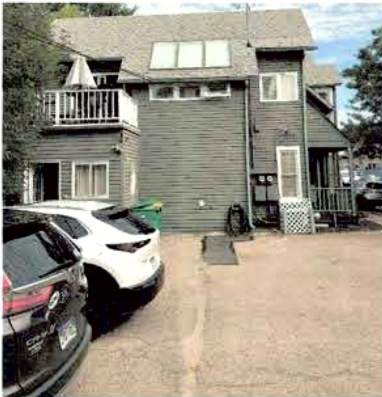
CURRENT PHOTOGRAPH SOUTH ELEVATION LOOKING NORTH
