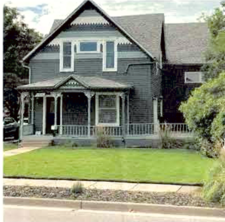
CURRENT PHOTOGRAPH NORTH ELEVATION LOOKING SOUTH
