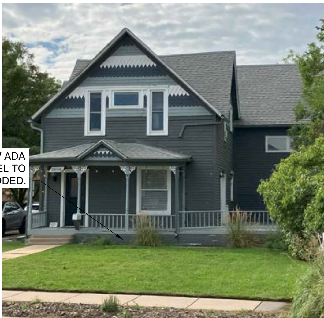
CURRENT PHOTOGRAPH NORTH ELEVATION LOOKING SOUTH
