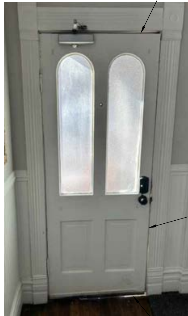
CURRENT PHOTOGRAPH EAST DOOR INTERIOR
