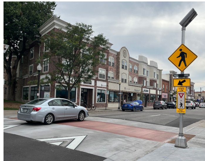
Rectangular Rapid-Flashing Beacon (RRFB) and raised pedestrian crossing on Main Street
