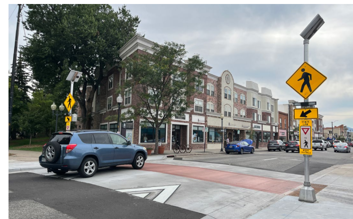
Rectangular Rapid-Flashing Beacon (RRFB) on Main Street
