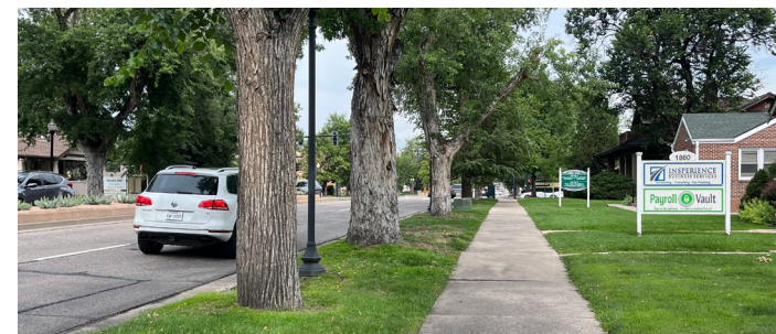
Detached sidewalk on Littleton Boulevard
