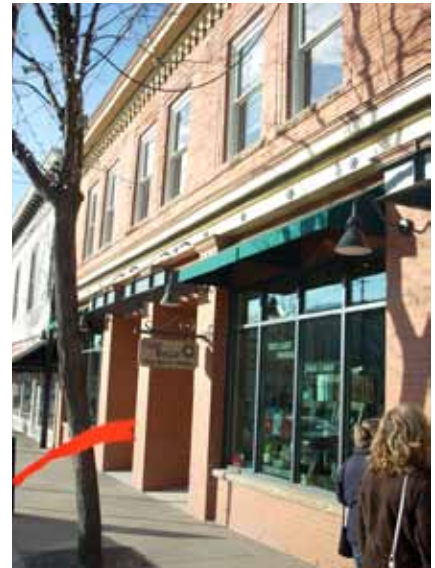
This contemporary but compatible storefront is an example of Approach C for replacing or reconstructing a historic feature.
