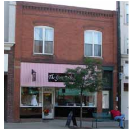
The building shown above is a rehabilitation opportunity. It retains many of its key features.
