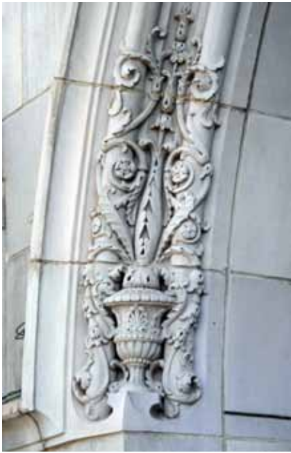
Preserve significant stylistic and architectural features.
