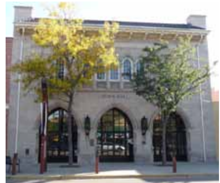
The Old Town Hall serves as an accent to the traditional commercial storefront framework of the historic district. The building has a row of three gothic arches defining the street level, with a wall of recessed doors and windows.
