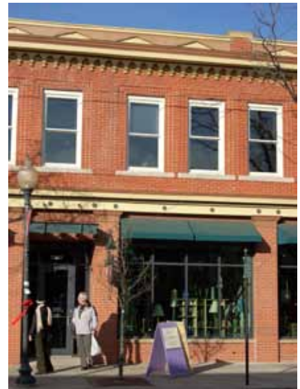
This commercial building in Downtown Littleton has many typical elements of a storefront (see diagram at left).
