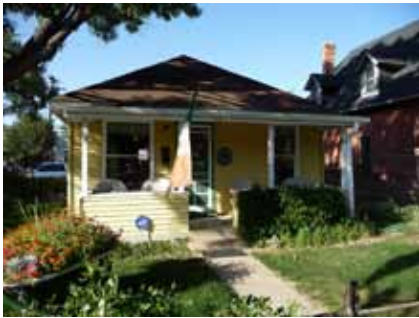
Certain areas retain a distinct historic residential character, defined by a landscaped front yard and side yard setbacks. Plantings and other landscape features should remain prominent in a historic residential setting.
