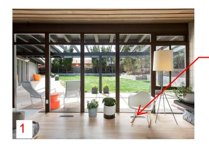
EXISTING FLOOR REGISTERS CONNECTED TO UNDERSLAB DUCT WORK
