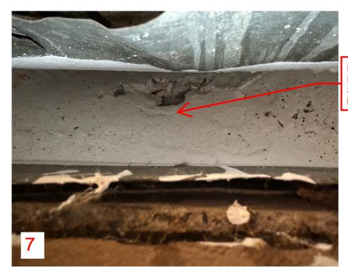
RUSTED THROUGH PORTIONS OF DUCT SEALED WITH LIQUID LATEX
