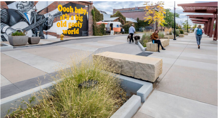
Image 34: Stormwater Planters with Curbs
