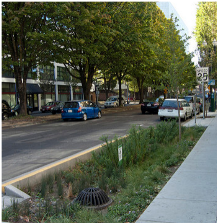
Image 13: Stormwater Planter with No Curbing or Walls
