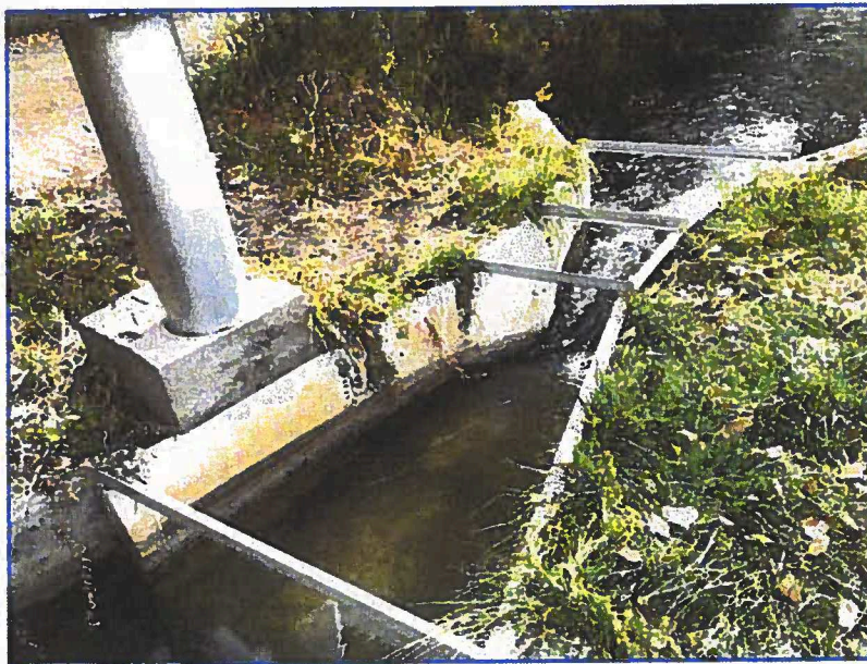
Figure 17: Parshall Flume located in the ditch just above its crossing of Big Dry Creek. Patented by Dr. Ralph L Parshall, a CSU professor in 1922, the invention made possible very accurate measurements of flowing water. Flumes of this type ended years of controversy over how much water was actually being used by ditch irrigators compared to their entitlement. Photo by author.
