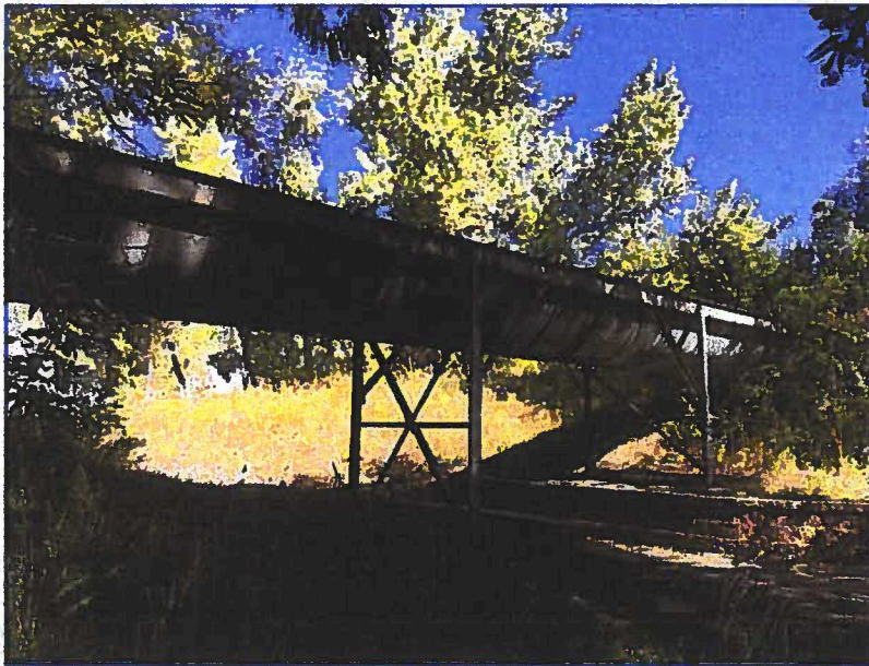
Figure 15 City Ditch Flume over Slaughterhouse Gulch in Littleton today. This is in Slaughterhouse Gulch Park, north of the Depot Arts Center. In the 1860's, before the arrival of the railroads in Denver, costs to ship structural iron from "the States" would have been prohibitive and the original structures of this type would have been made of wood. It has been speculated that this particular structure dates from the mid-1940's. Photo by author.
