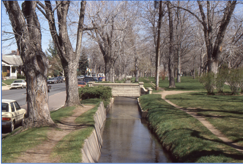
Figure 10: The City Ditch in Denver's Washington Park today. South Downing Street on left. Washington Park and the City Ditch there were listed on the National Register of Historic Places in 1976. Today, the irrigation water in the City Ditch in Washington Park continues to flow north in a pipeline in the Ditch's original alignment to fill the lakes at the Denver Country Club and City Park. The water from those lakes is then pumped into sprinkler systems to irrigate those historic green spaces. The actual water in the Ditch is reclaimed water from the Metro Wastewater facility which has been treated to a high level. It is a wise use of a scarce resource in our arid climate.
