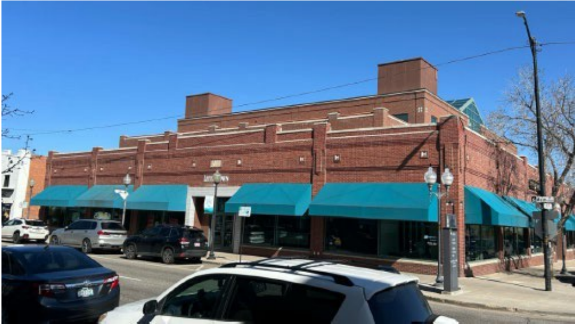
Figure 3: View of existing south facing façade at 2329 W. Main Street.
