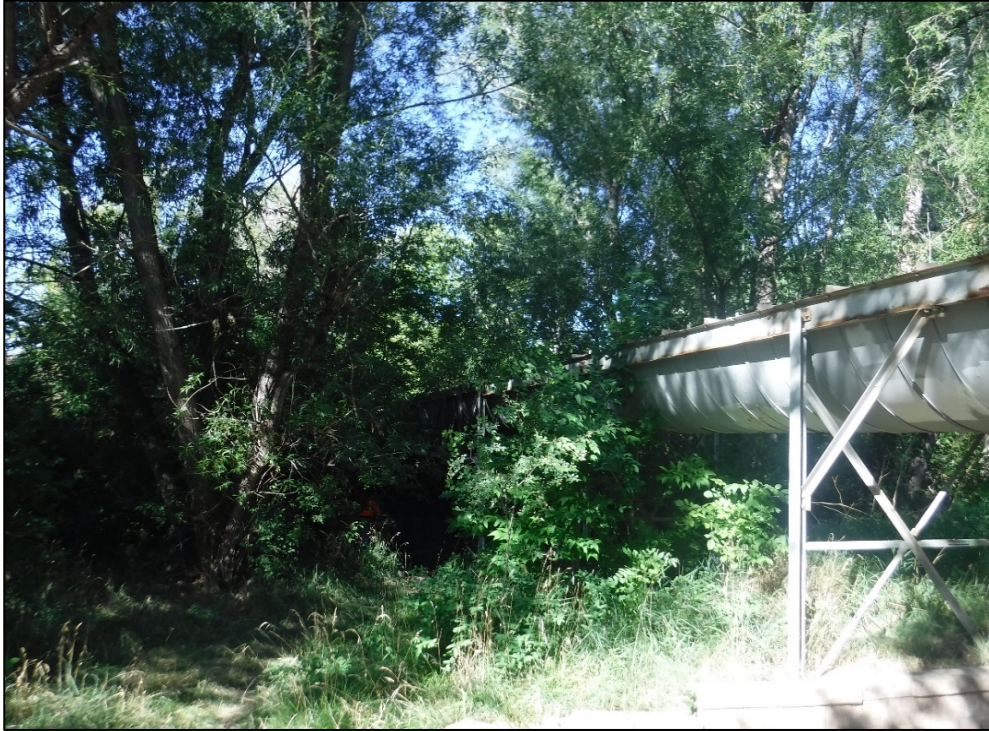
Elevation looking southwest.
