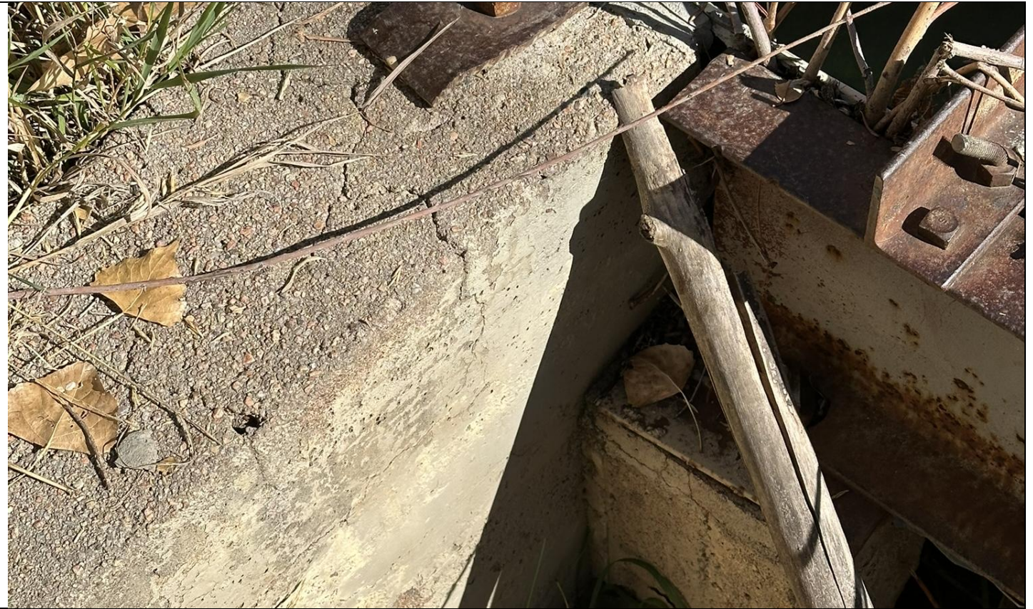
The wingwall. Negative
