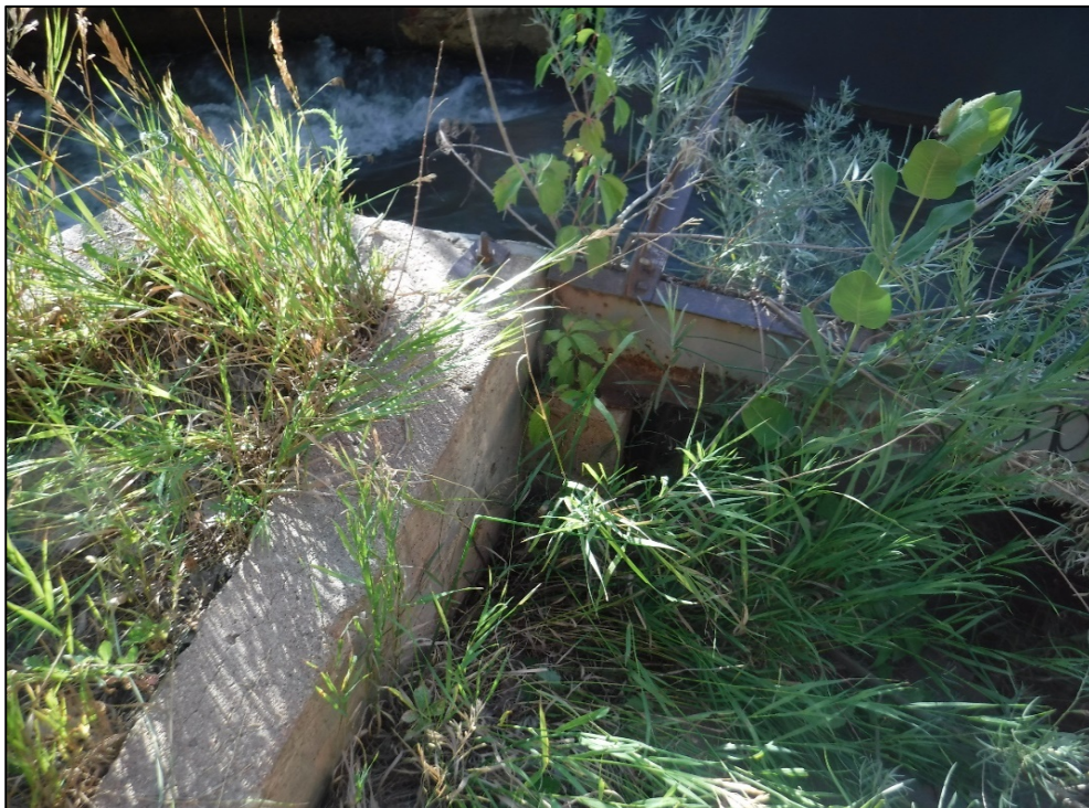
Northwest end of structure with vegetation growth.
