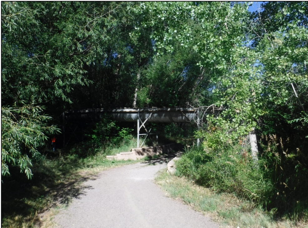
Elevation looking west (Spans 8, 9, and 10).
