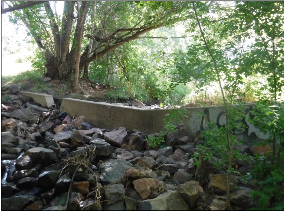
Concrete weir across channel under Span 6.
