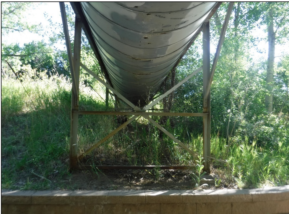
Pier 10 trestle general.
