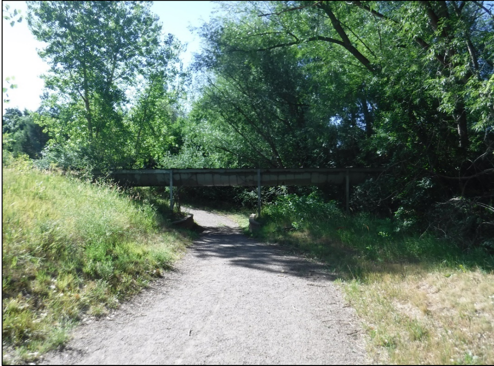
Elevation looking east (Spans 8, 9, and 10).
