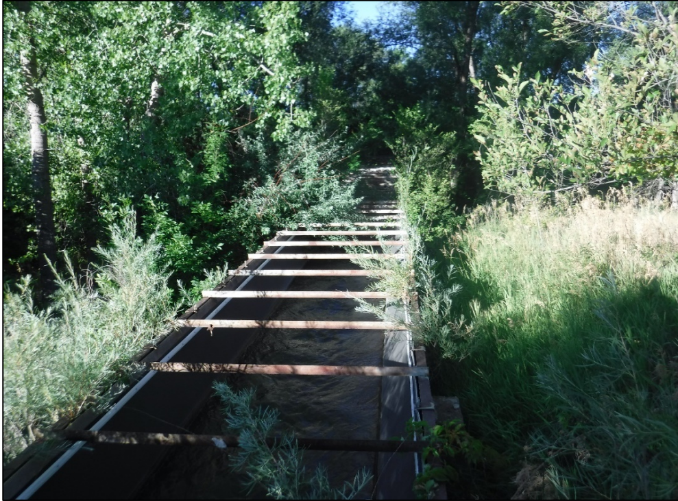
Flume looking southwest (topside).
