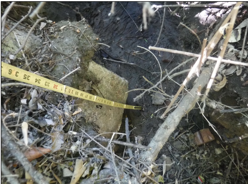
Pier 6 east footing south face fully exposed with no undermining.
