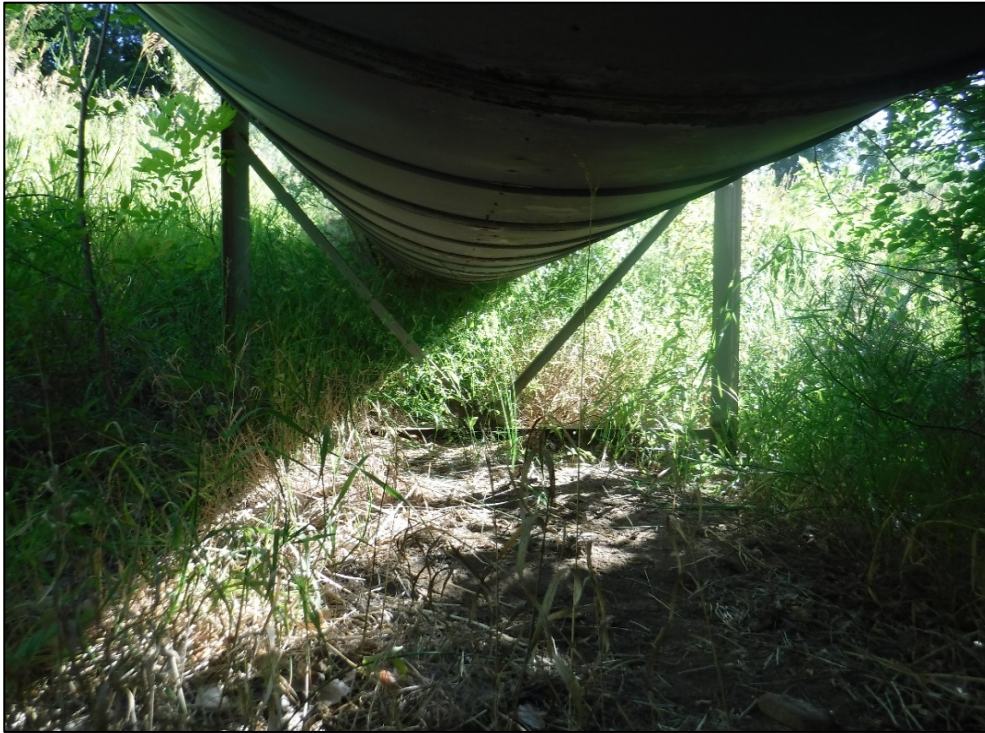
Pier 12 trestle general.
