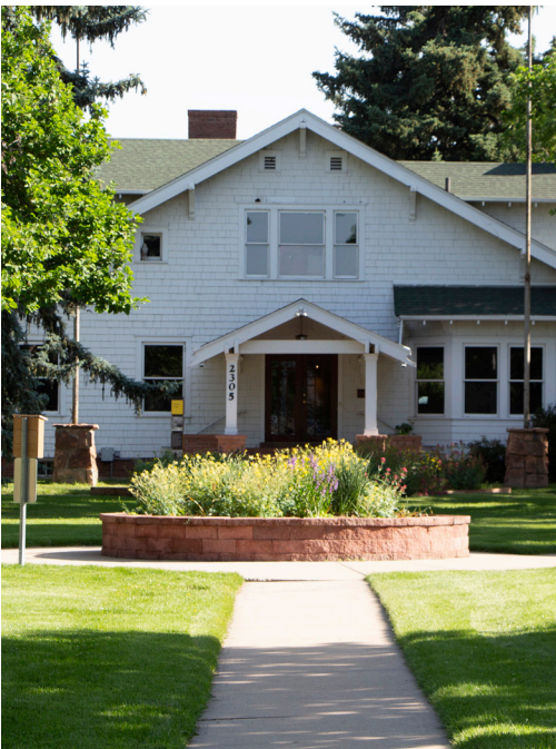
View of paved entry to Geneva Lodge.
