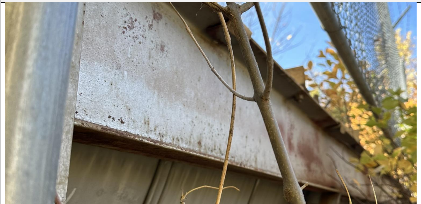
Close-up of a girder. Negative
