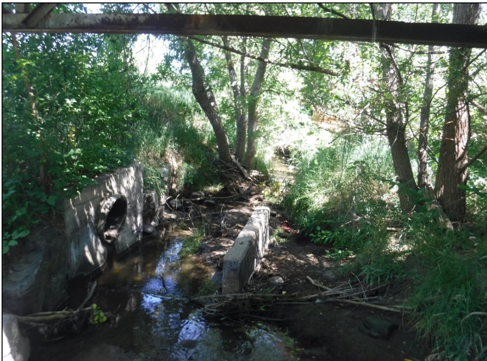
Channel looking north downstream.
