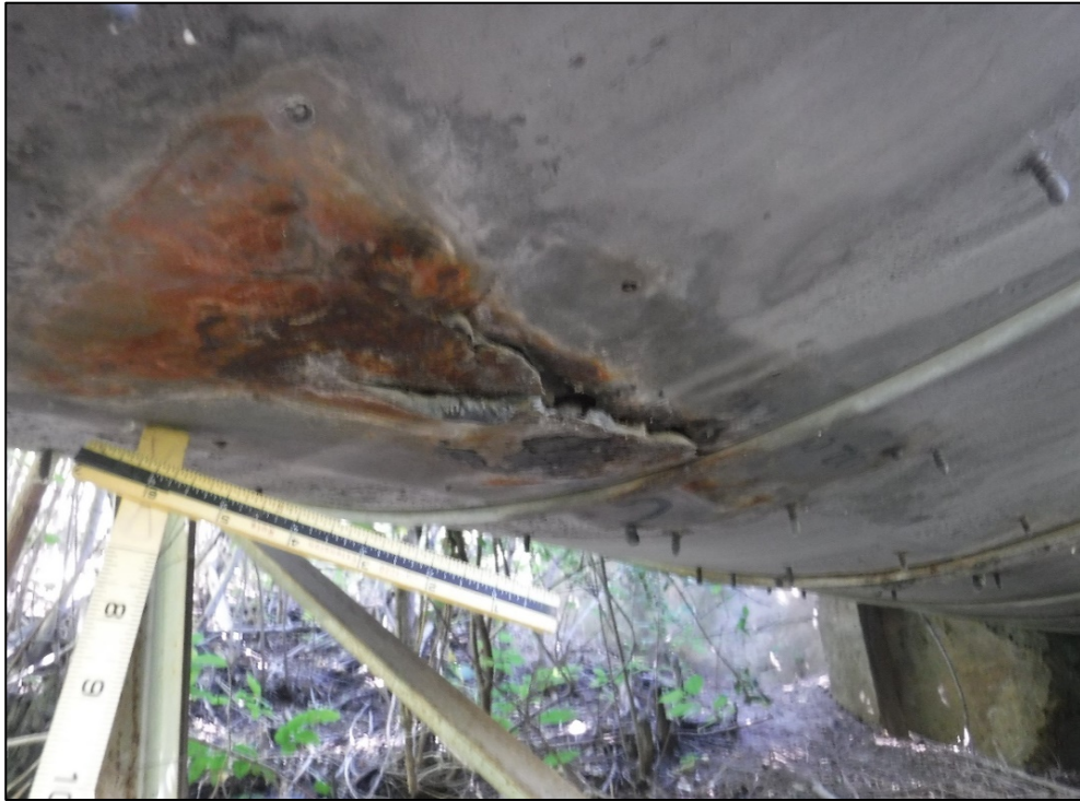
Span 2 near Pier 2 has area of tear and damage.
