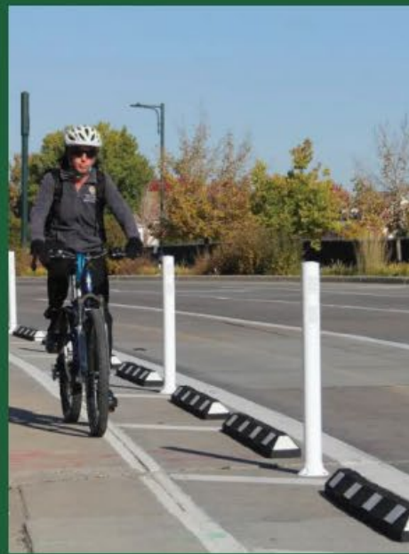
Example of rubber parking stops and delineators
