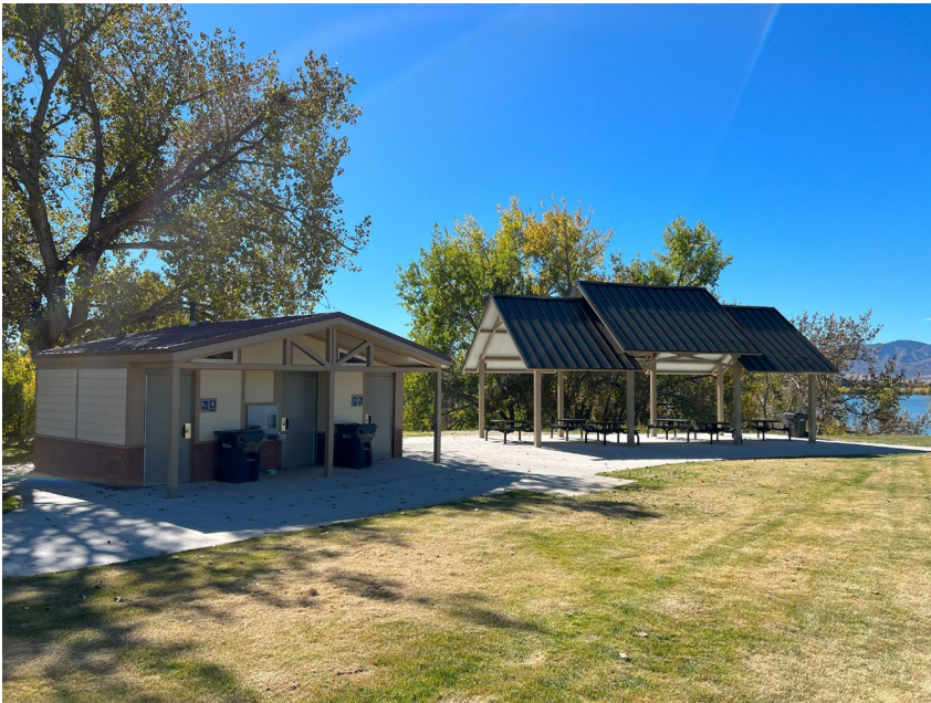
Writers Vista Restroom and Shelter
