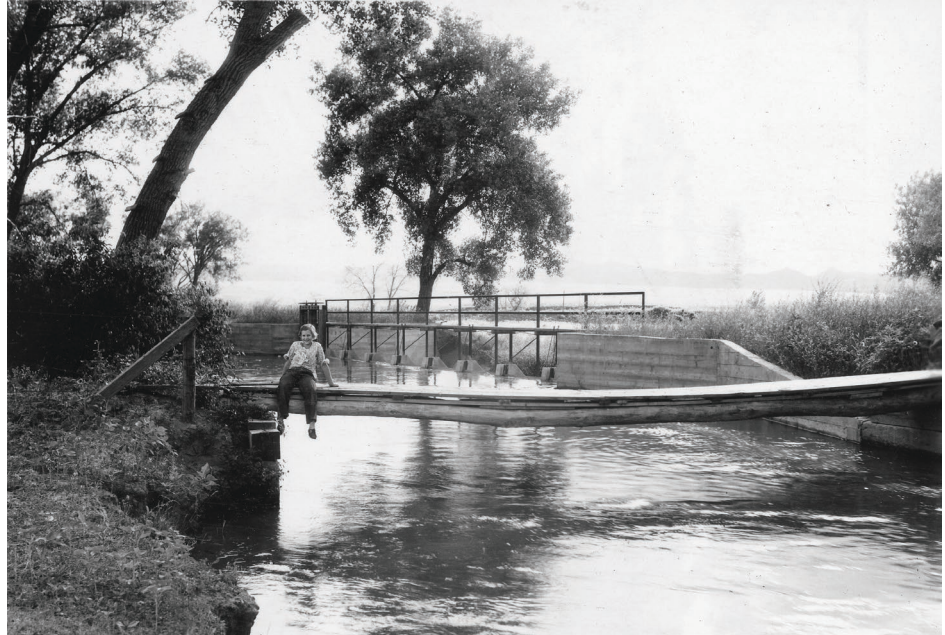
High Line Canal Gates at Big Dry Creek
