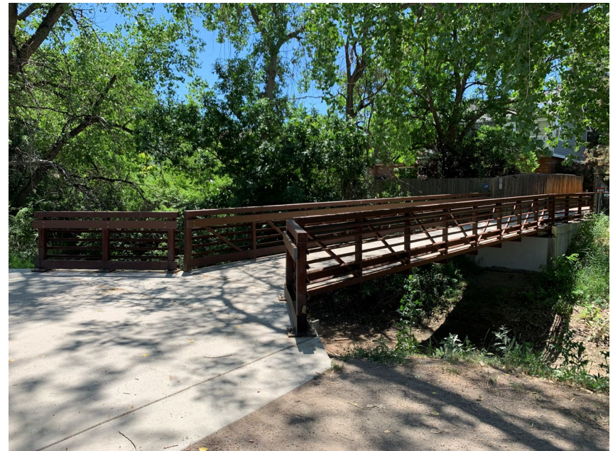
Bannock Street Ped Bridge
