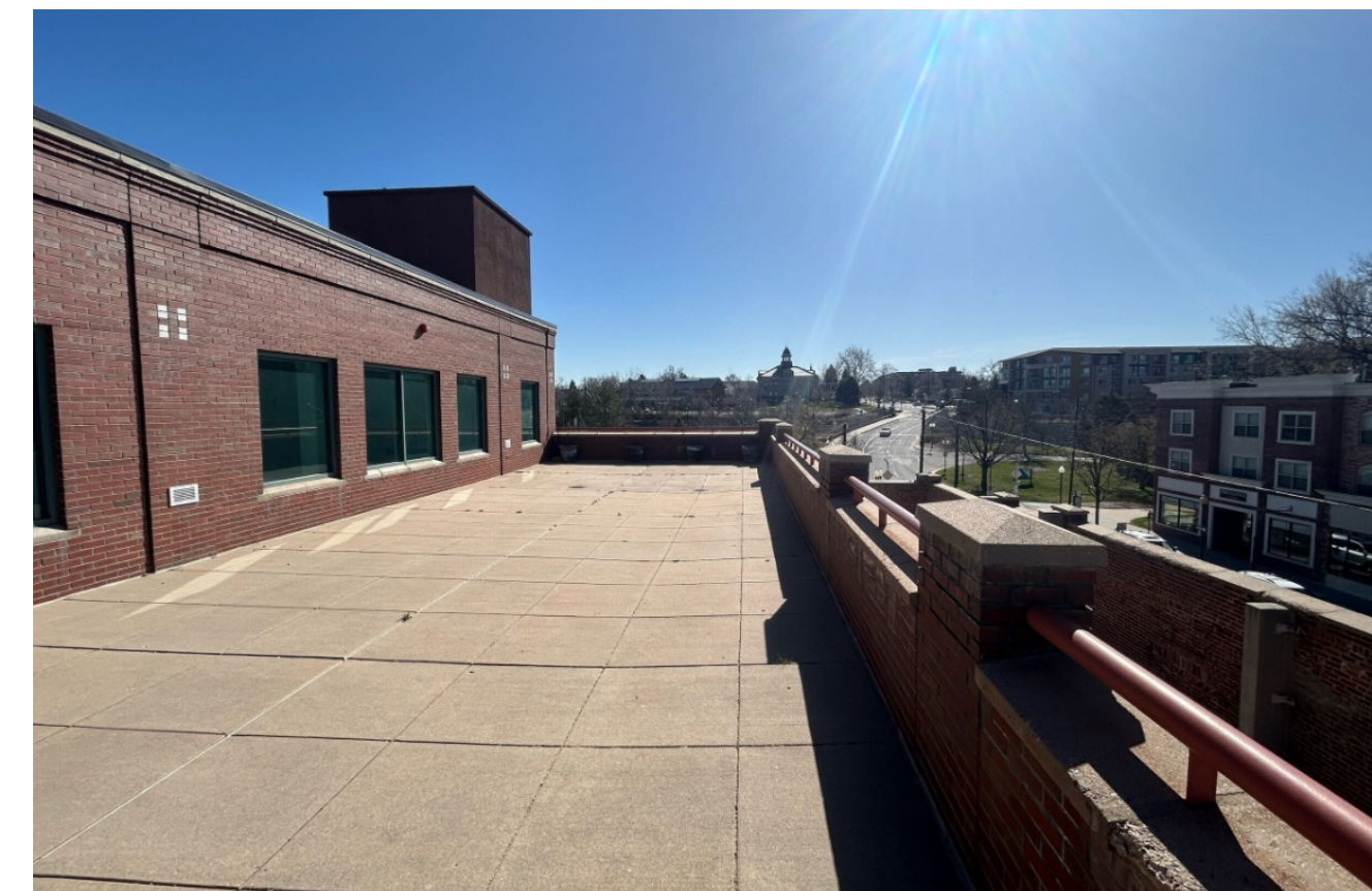
VIEW ON ROOF LOOKING EAST
