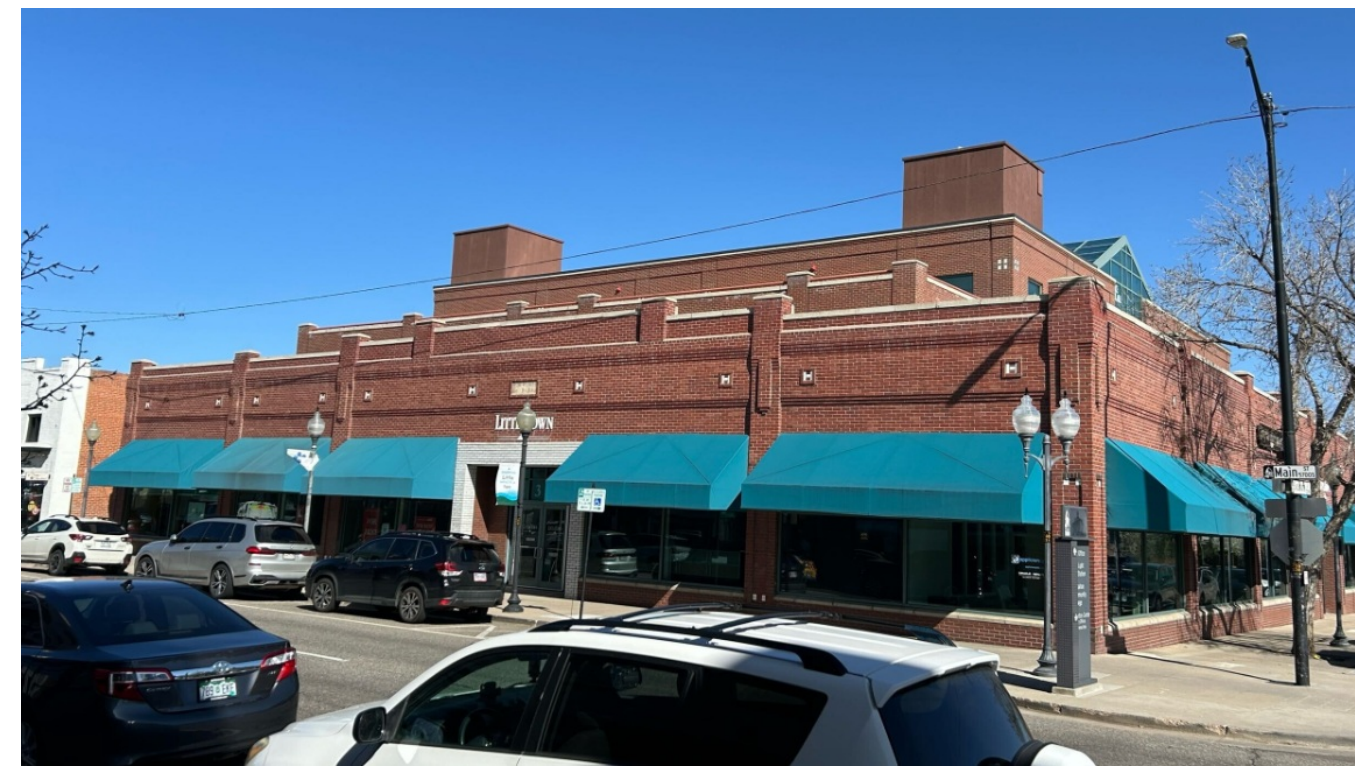
VIEW FROM MAIN ST.
