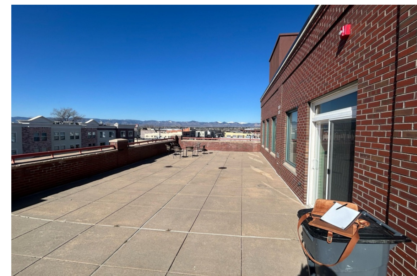
VIEW ON ROOF LOOKING WEST
