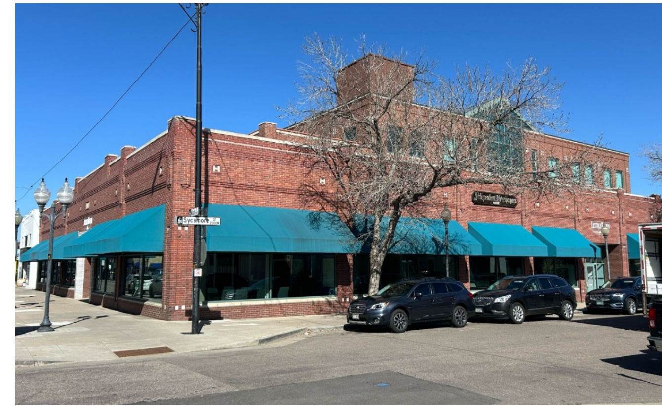
VIEW FROM SYCAMORE ST.
