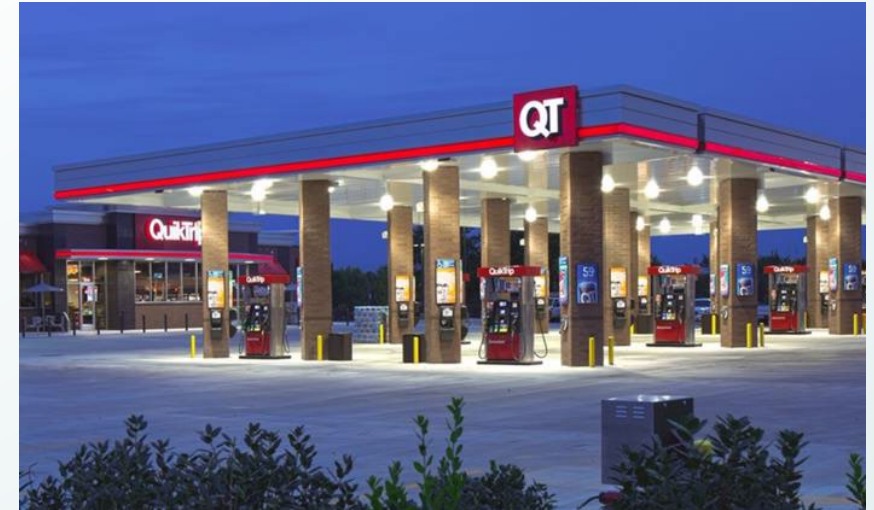
Newly constructed QuikTrip off Belleview and Santa Fe
