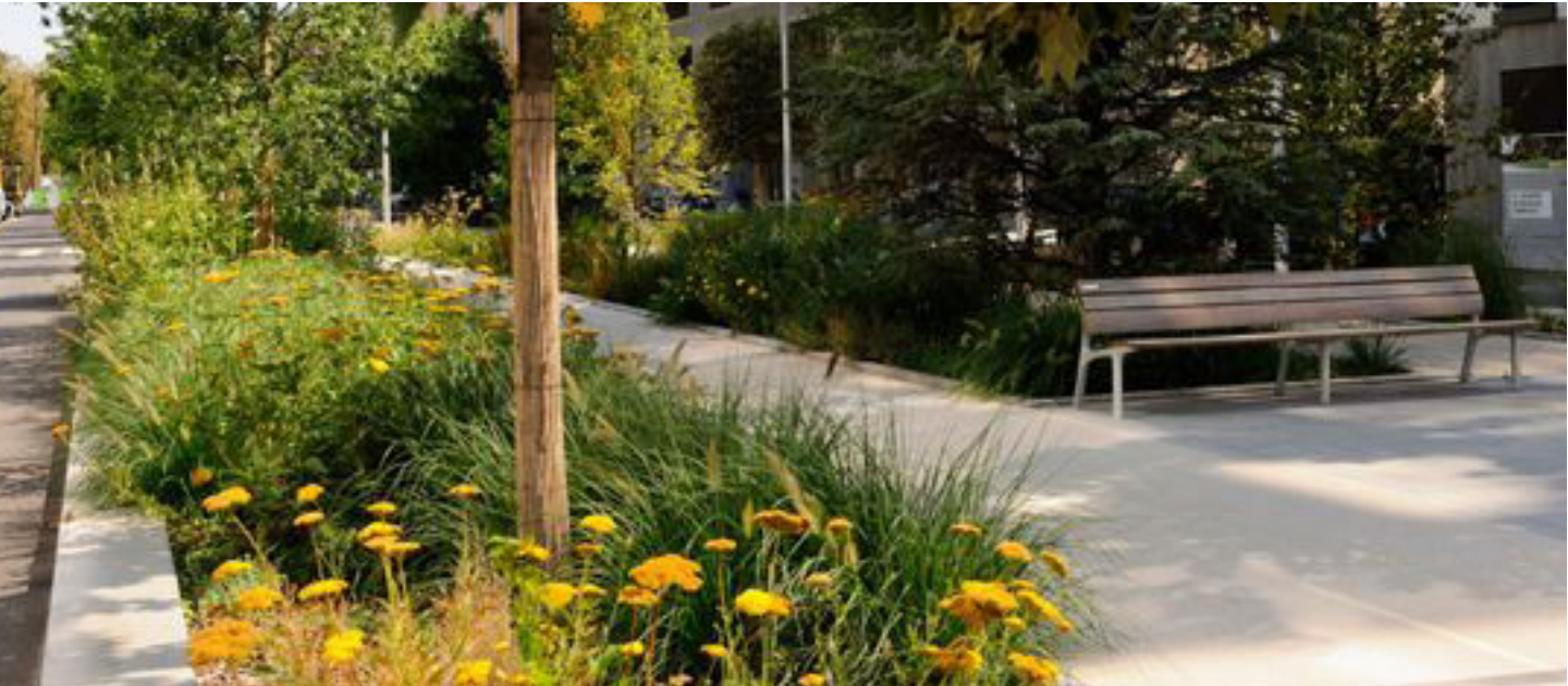
Image 9: Flow Based Treatment Planter Accepting Runoff from Sidewalk Only
