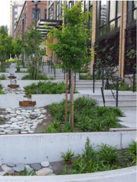
Image 23: Stormwater Planters with Weir Walls
