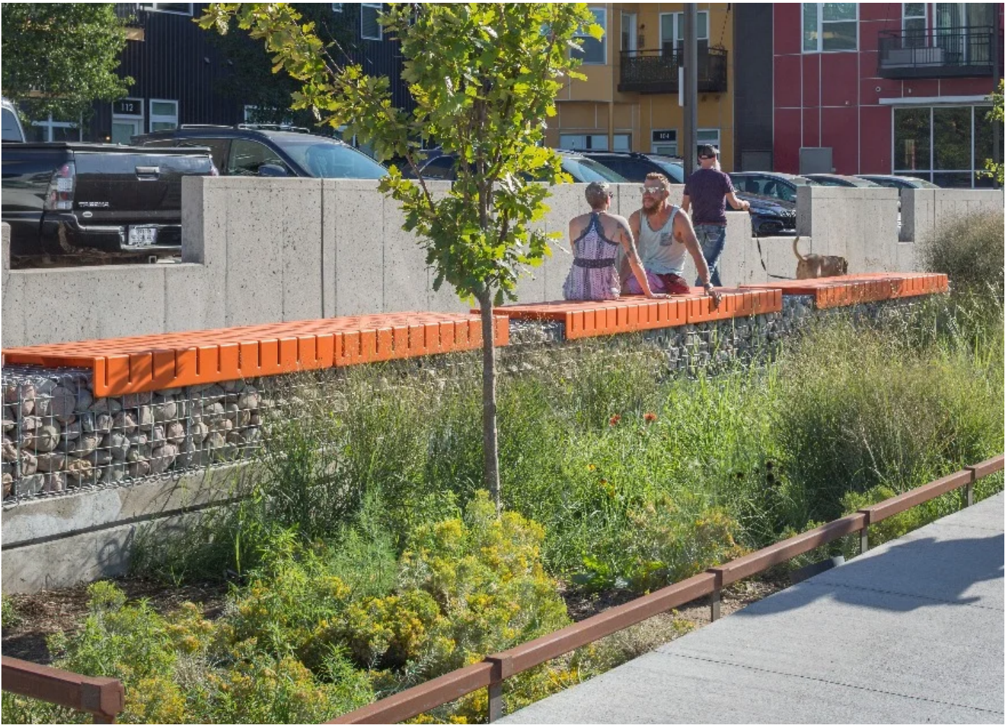
Image 26: Sunken Stormwater Planters with Gabion Seat Walls and Kick Rails
