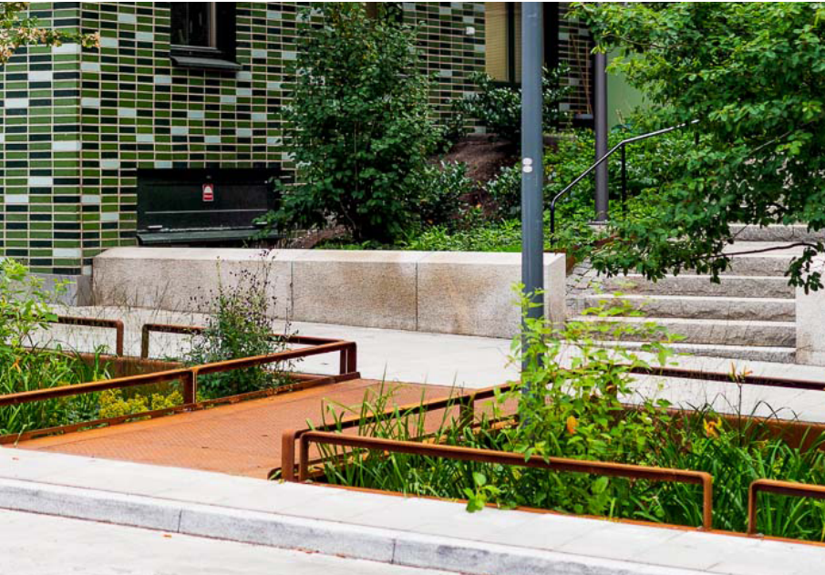
Image 16: Sunken Infiltration Planters Treat Stormwater
