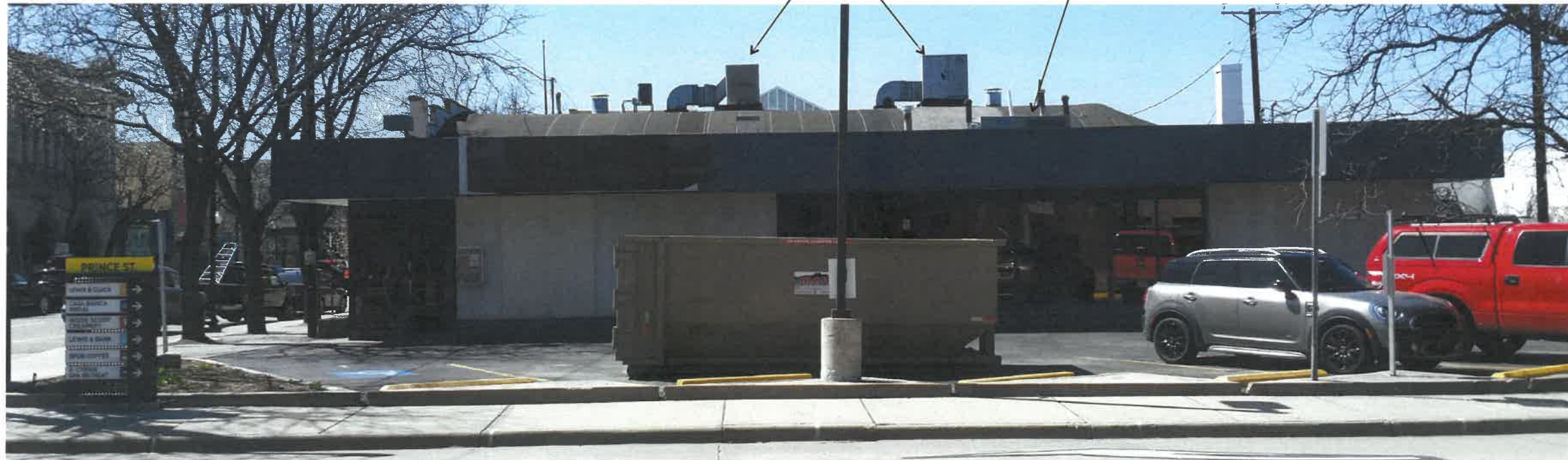
3 EXISTING EAST FACADE NTS
