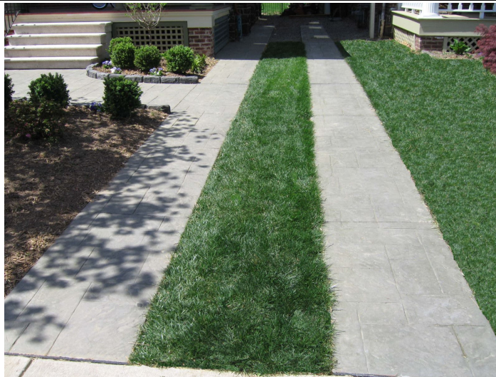
Figure 10-1-3.7.B.2 Wheel Strip Driveway Example
