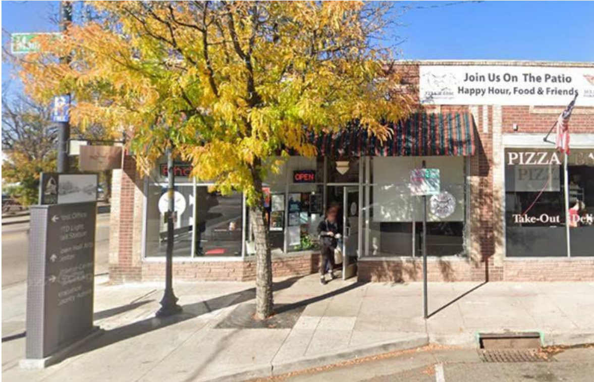
Figure 3: View of existing south facing façade at 2399 W. Main Street.
