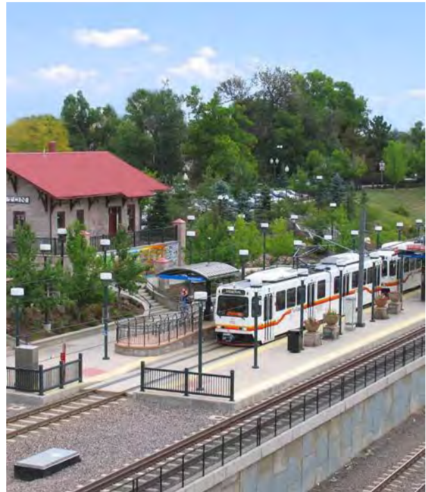
RTD's Downtown (above) and Mineral light rail stations are increasingly important as regional connections.
