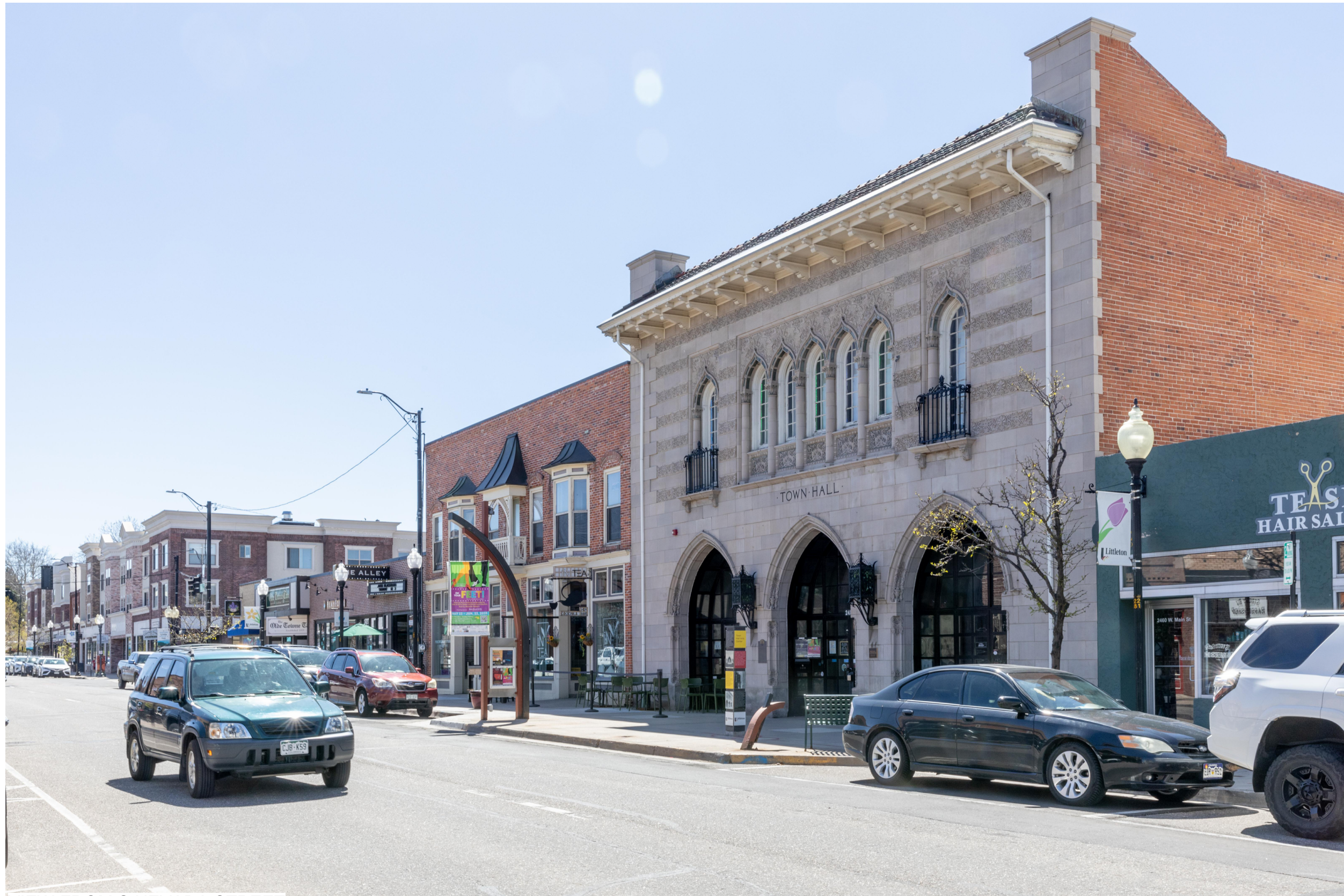
VIEW FROM S NEVADA STREET
