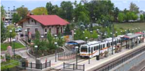
The Denver and Rio Grande Railroad Depot has returned to its use as a passenger station for those utilizing the Southwest Corridor light rail line.
