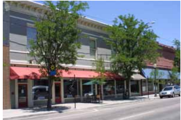
The façade restoration work on the Batschelet Building on Main Street was completed in 1995 and contributes to downtown's historic small town character.
