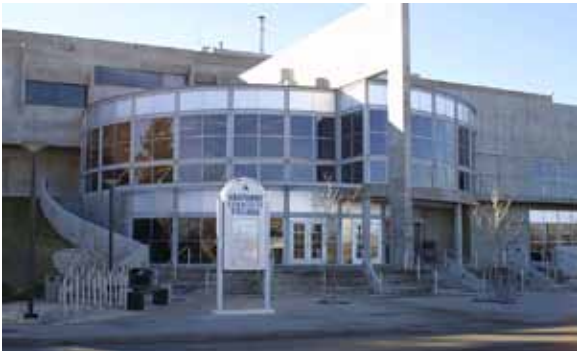
Arapahoe Community College is located at the southern end of the Downtown Neighborhood and has 18,000 students and 700 faculty and staff.
