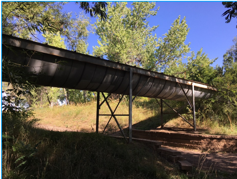
Figure 12: City Ditch Flume over Slaughterhouse Gulch in Littleton today. This is in Slaughterhouse Gulch Park, north of the Depot Arts Center. In the 1860's, before the arrival of the railroads in Denver, costs to ship structural iron from "the States" would have been prohibitive and the original structures of this type would have been made of wood. It has been speculated that this particular structure dates from the mid-1940's. Photo by author.
