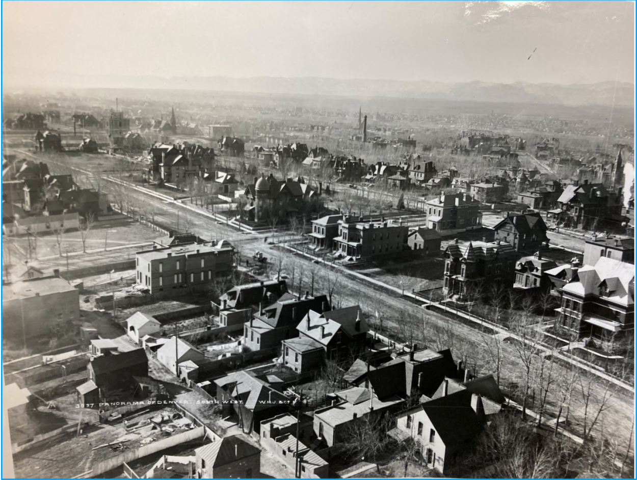
Figure 6: This Denver street scene taken by W. H. Jackson is likely from the mid 1870's to early 1880's, based on the estimated age of the young trees. A careful examination shows lateral irrigation ditches adjacent to the street with rows of young trees between the street and sidewalk. Note that individual homes have a bridge over the ditch to allow access to a carriage in the street. The ditch water would have stimulated the trees to grow in the arid climate.
