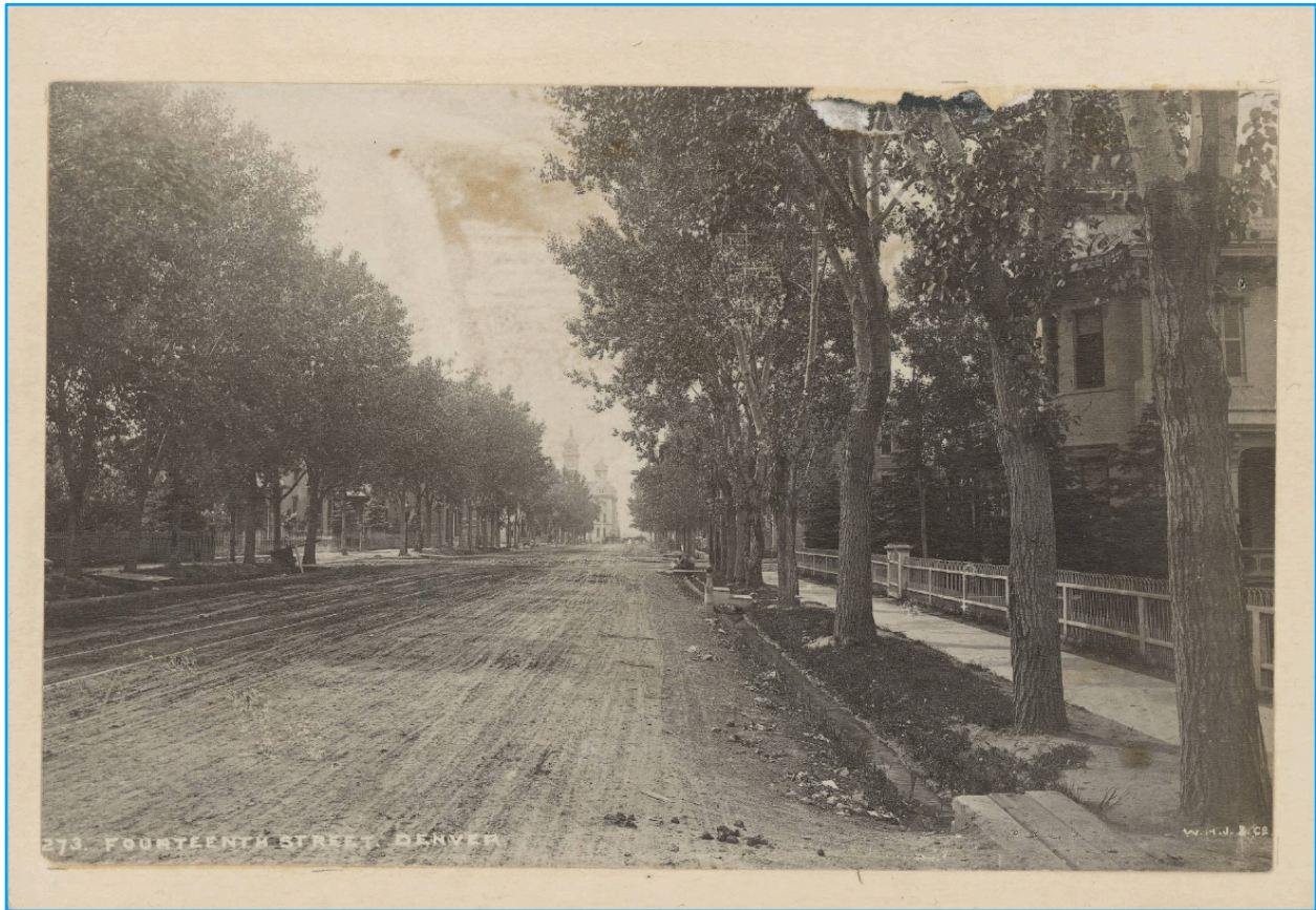
Figure 7: Fourteenth Street Denver circa 1880's. Note the small lateral ditch with water at lower right and the footbridges across it, including one with steps to make it easier to board a carriage. The mature trees show the positive effect the irrigation water had for their survival and growth.
