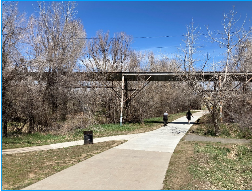
Figure 15: City Ditch Flume over Big Dry Creek in Englewood today. The paved trail shown in the photograph along the Creek connects the Highline Canal Trail in Greenwood Village with the Mary Carter Greenway Trail along the South Platte River.
