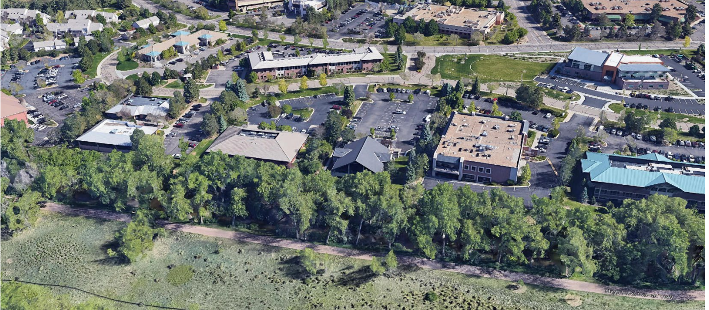
Section of SouthPark business park in south Littleton, with office uses and parking areas nestled amid generous landscaping and buffers, and with the High Line Canal Trail adding to the Suburban character.
