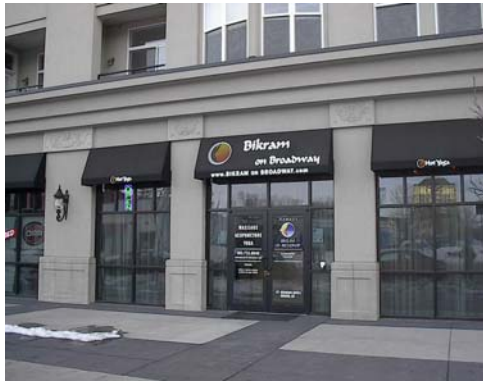
Example of extensive undesirable text on sloped portion of awnings Illustration 5.5.7.g6
