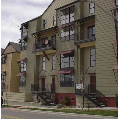
Example of acceptable metal awnings Illustration 5.5.7.g7a
