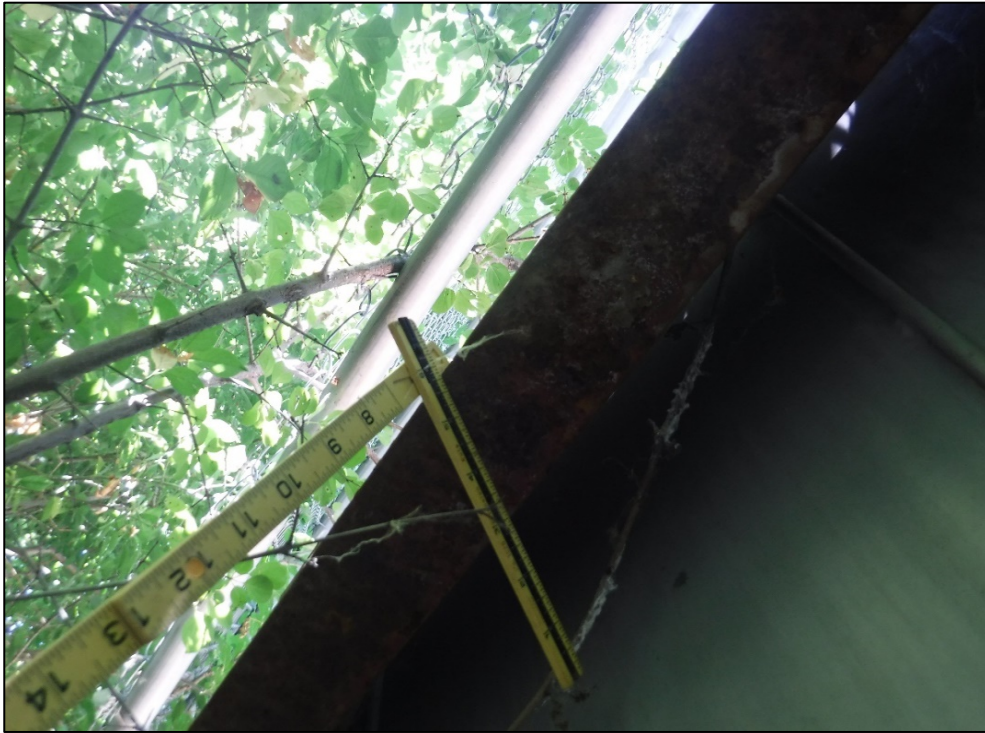
Beam has R1 corrosion, typical.
