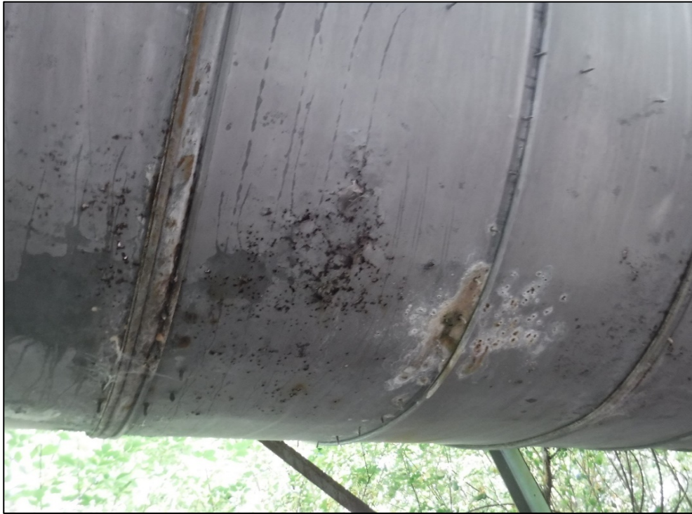
Span 4 underside has area of perforation through liner with rust stains.
