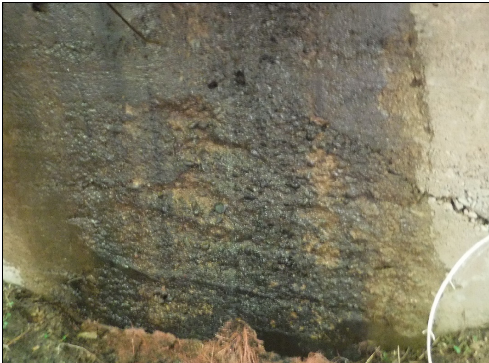
Abutment 6 has S3 scaling.
