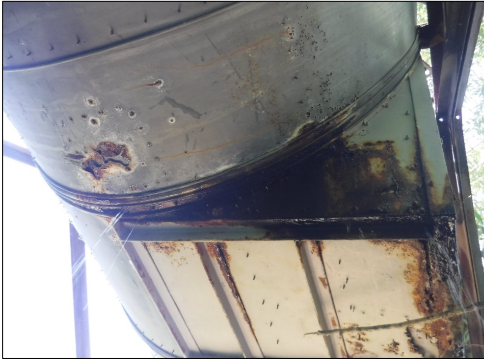
Span 3 at joint has R4 corrosion holes with active leakage.
