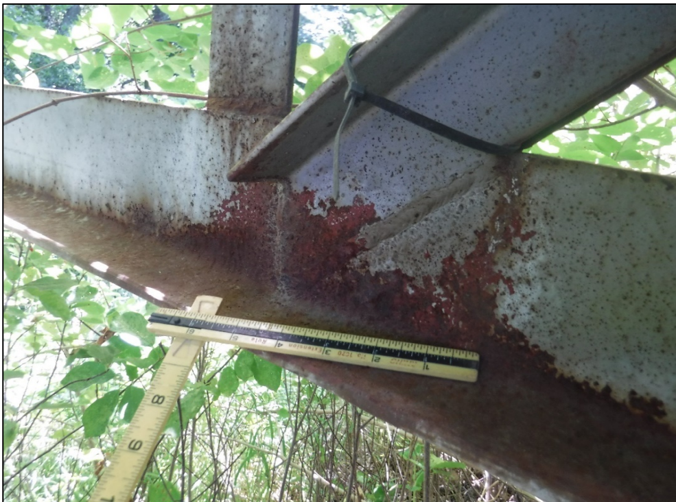
Truss 3A lower chord has R1 corrosion, typical.
