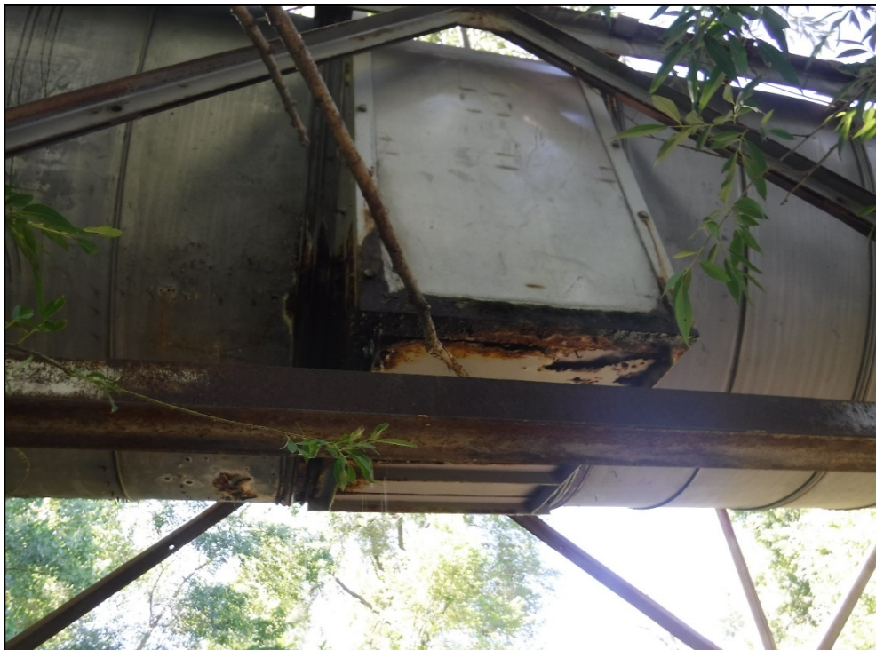
Span 3 active leakage at diversion with R4 corrosion holes.
