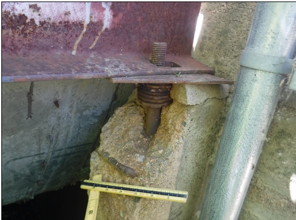
A1 north end spall with exposed rebar and anchor and missing nut at bearing.
