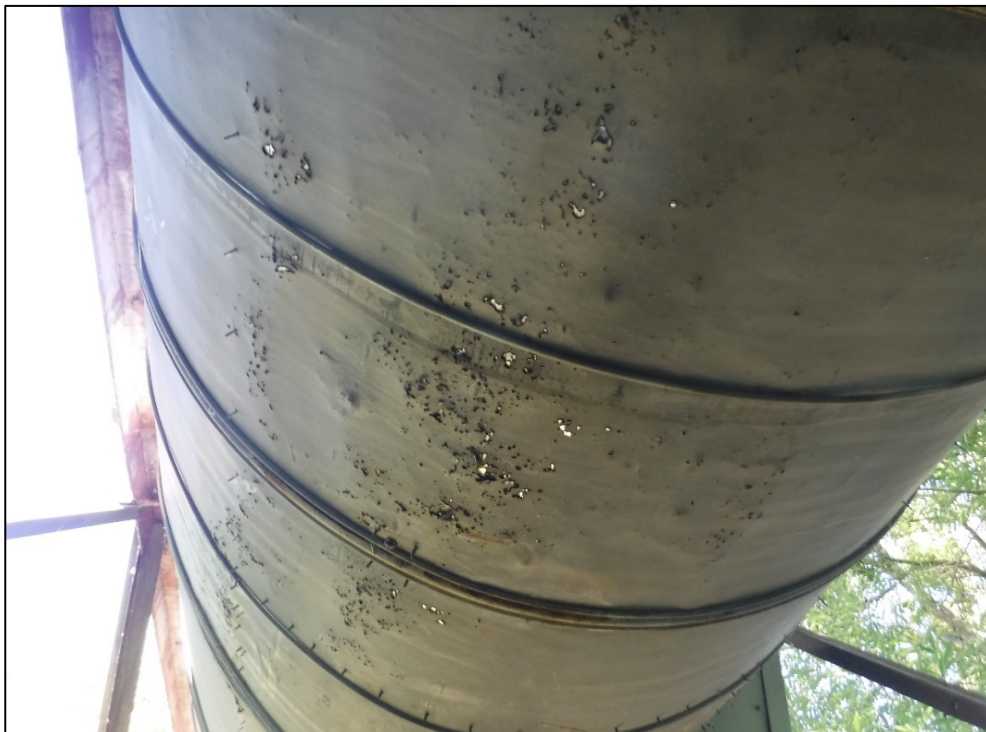
Span 3 deck underside has area of perforations through liner.
