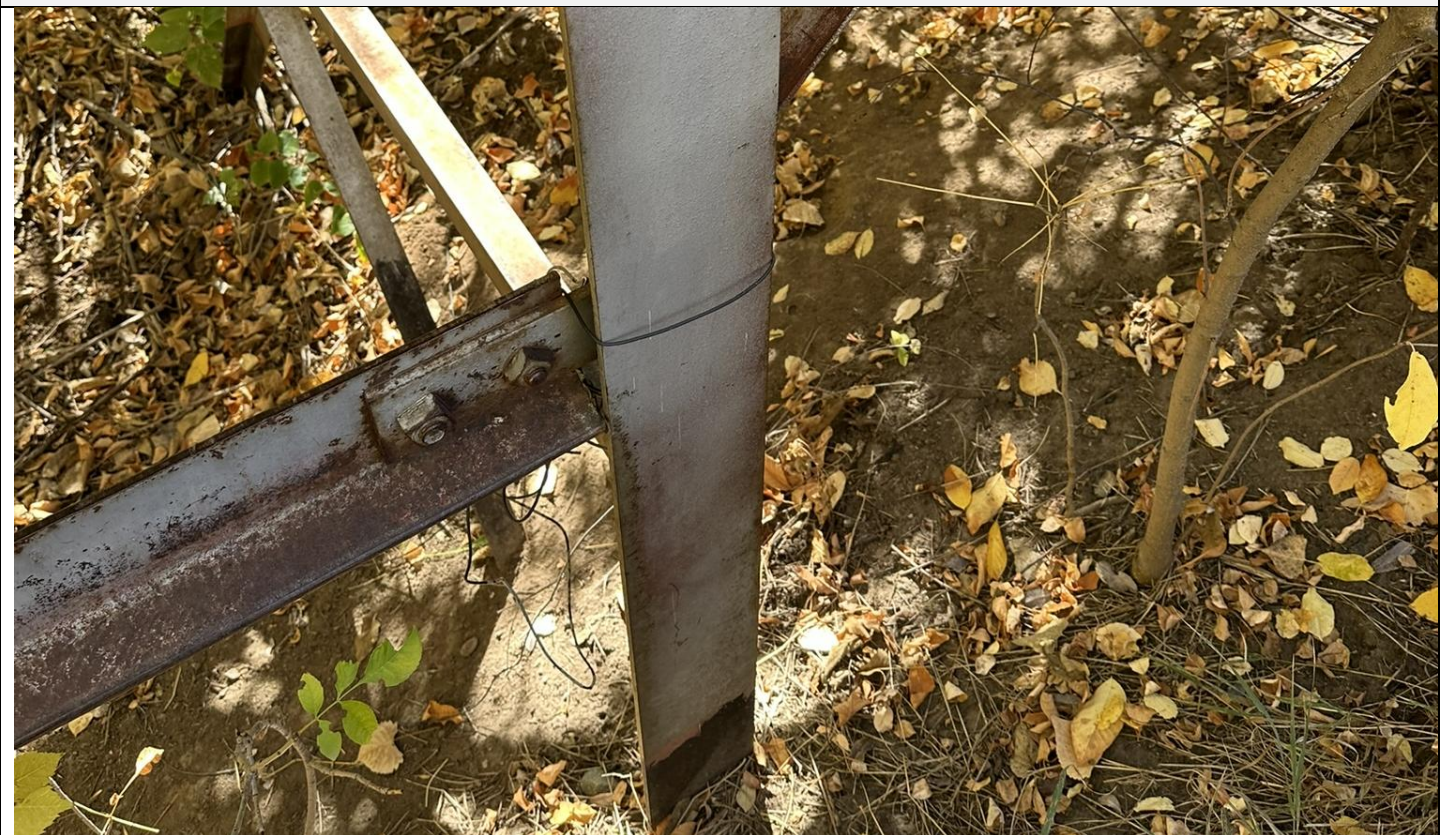
The vertical supports are identified as Towers in this report; the towers on this flume had two types of paint, silver and black. The black paint is only present on the West end of the tower, near and under the ground.
