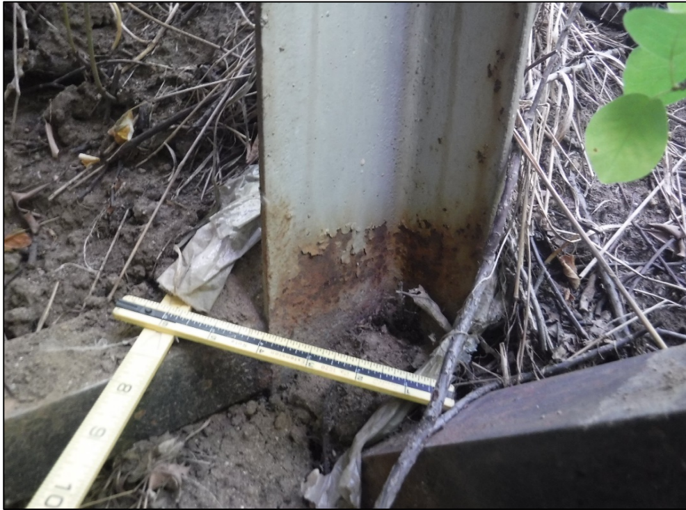
Trestle vertical at groundline has R1 corrosion, typical.
