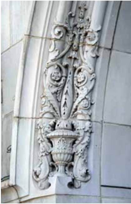
Preserve significant stylistic and architectural features.
